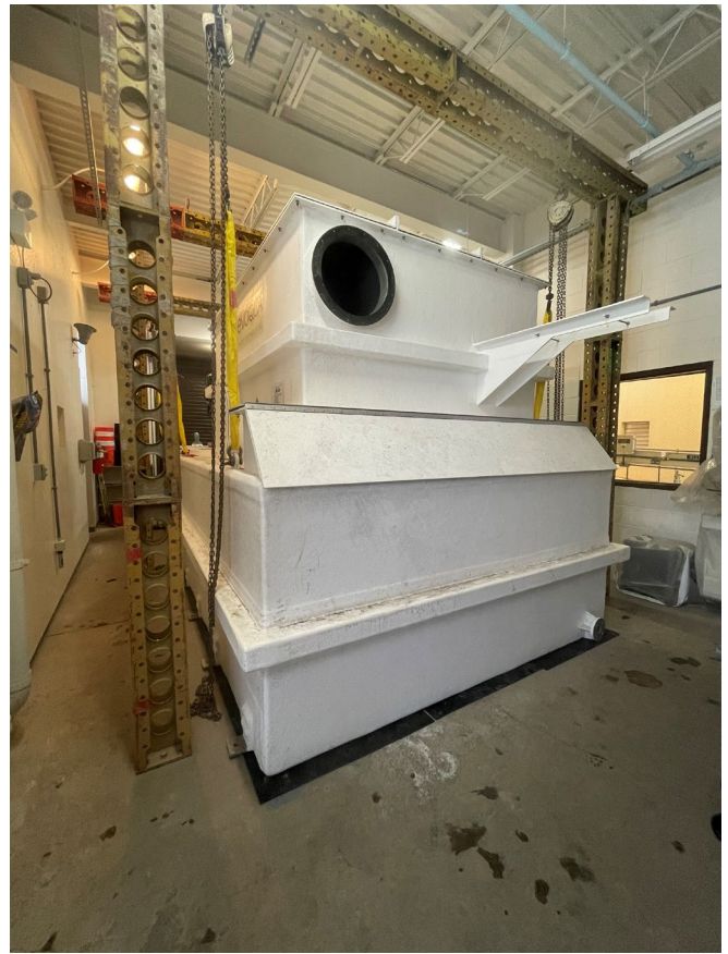
2021 Chlorine Scrubber Improvements Project Positioning the New Chlorine Scrubber in Building 75
