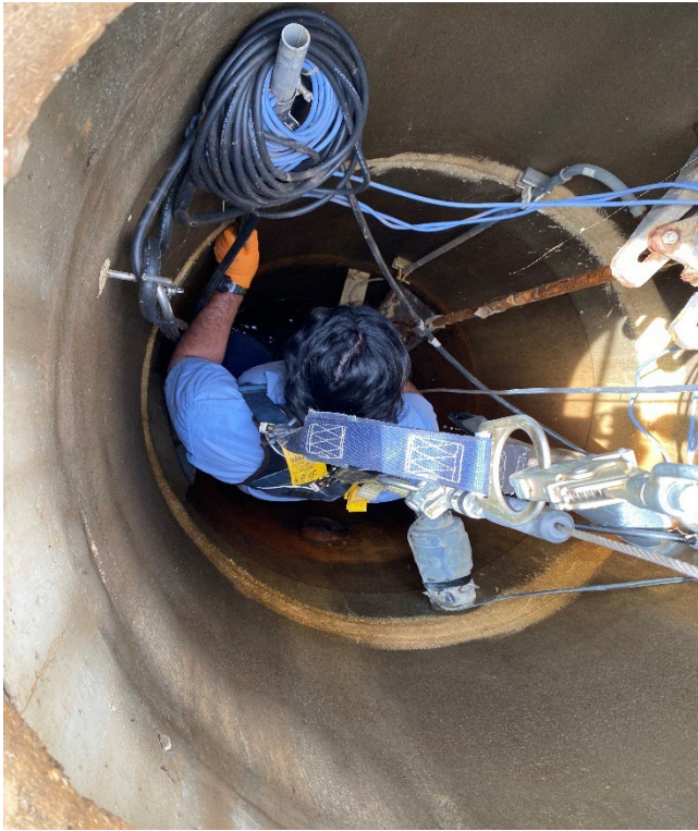
Odorous Air Sump Float Repair
