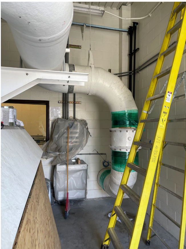
2021 Chlorine Scrubber Improvements Project Installation of the New Chlorine Scrubber Ducting
