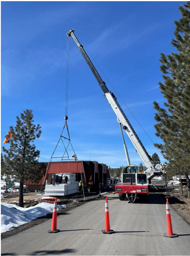
2021 Chlorine Scrubber Improvements Project Installation of the New Chlorine Scrubber
