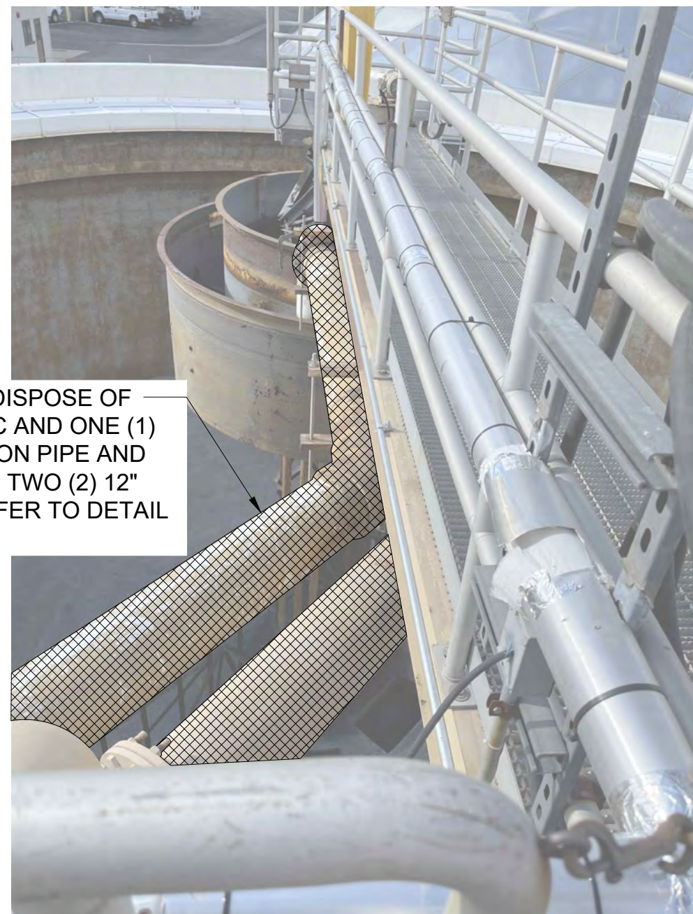
PIPE REPLACEMENT P-32 SCALE: NTS 57-M-103
