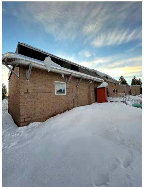
2020 Headworks Improvements Project Project Nearing Final Completion
