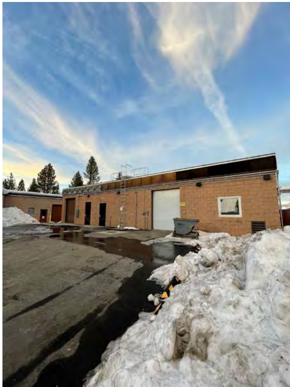
2020 Headworks Improvements Project Project Nearing Final Completion
