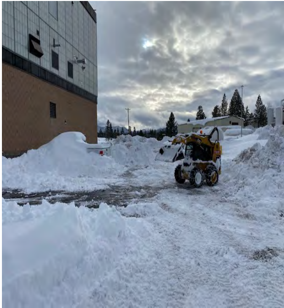
Snow Removal near Dewatering
