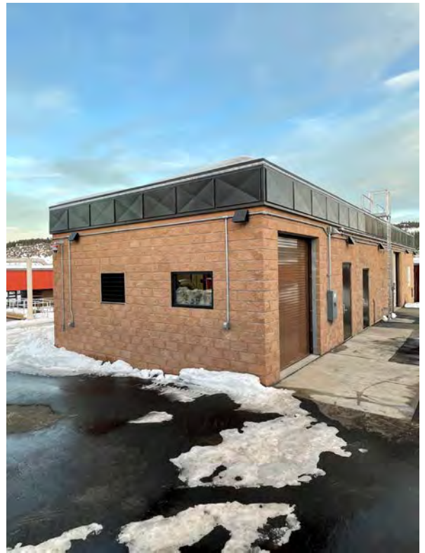
2020 Headworks Improvements Project Project Nearing Final Completion
