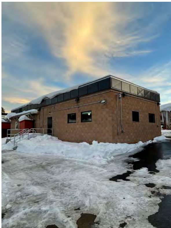
2020 Headworks Improvements Project Project Nearing Final Completion
