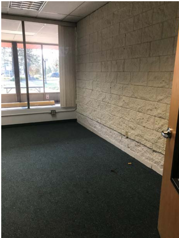
2020 Admin. Building Remodel Project - Before
