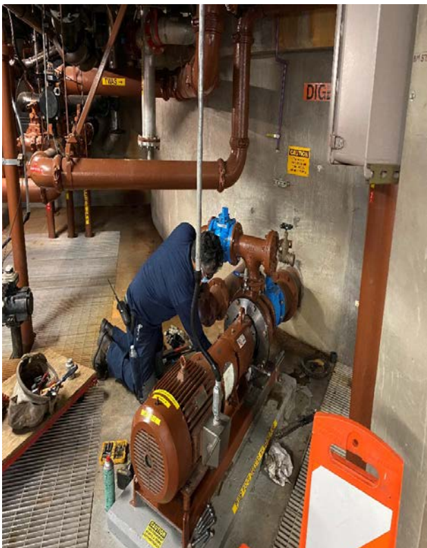
Sludge Recirculation Pump Rebuild
