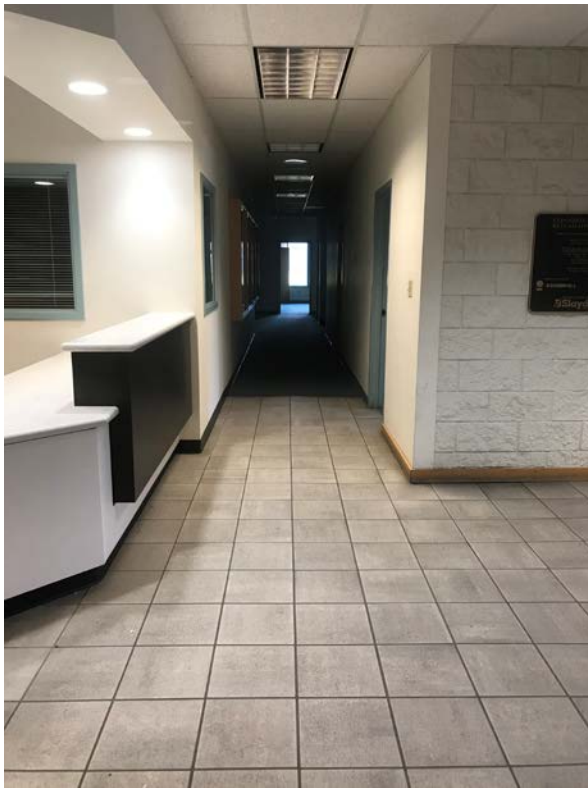
2020 Admin. Building Remodel Project - Before
