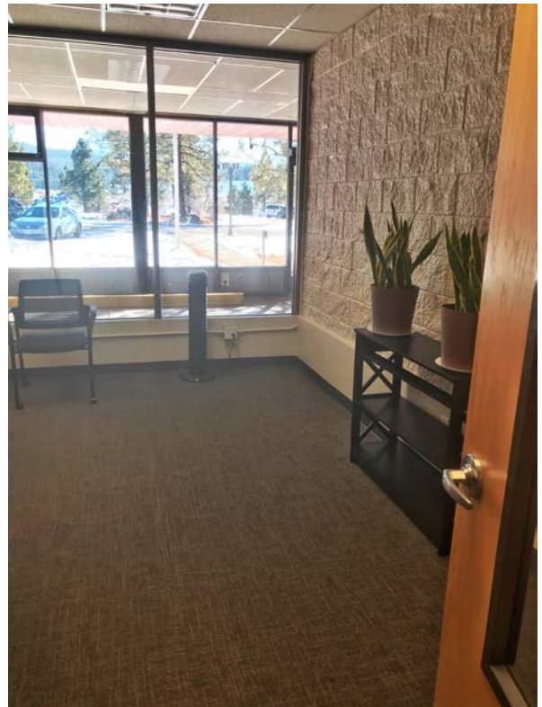
2020 Admin. Building Remodel Project - After
