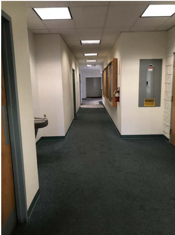
2020 Admin. Building Remodel Project - Before
