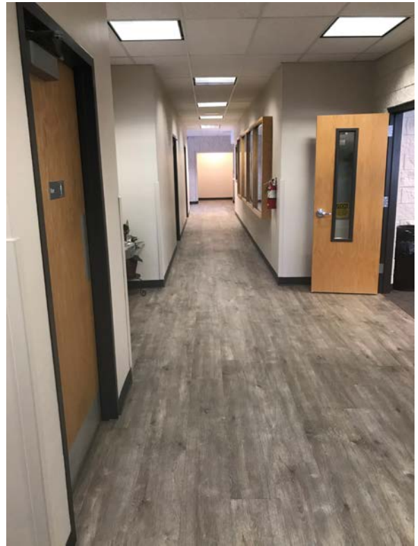
2020 Admin. Building Remodel Project - After
