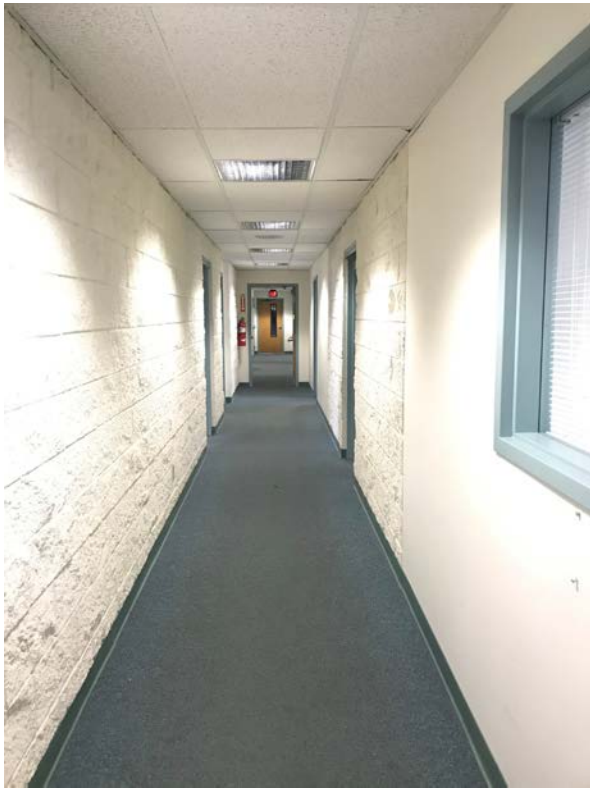
2020 Admin. Building Remodel Project - Before
