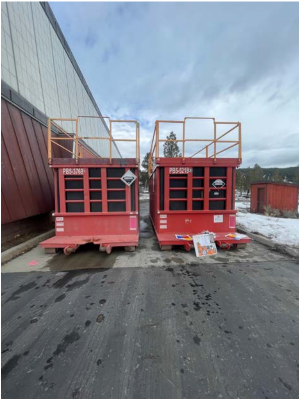
2022 Sodium Hypochlorite Disinfection Project Rental Tanks Offloaded
