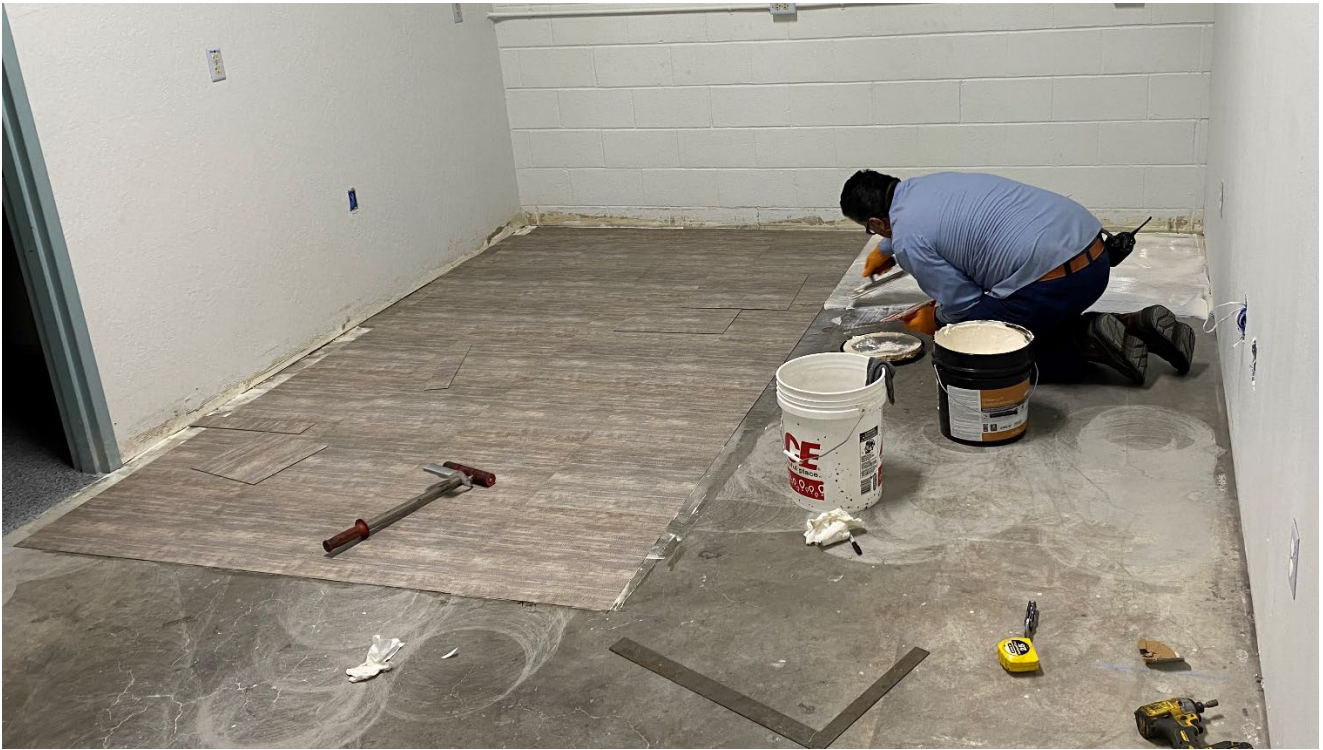
Flooring Installation in E&I Office
