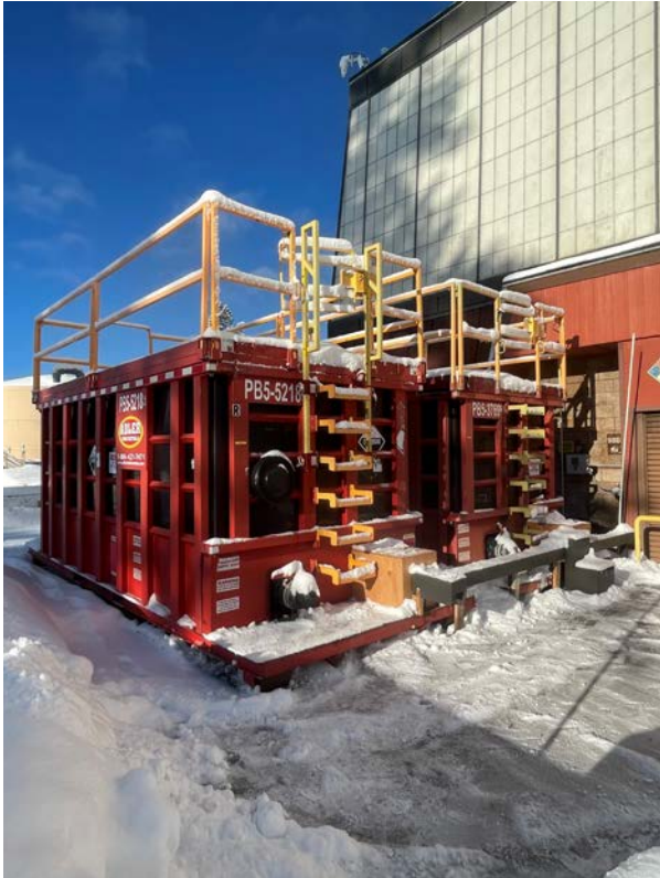
2022 Sodium Hypochlorite Disinfection Project Rental Tanks Connected
