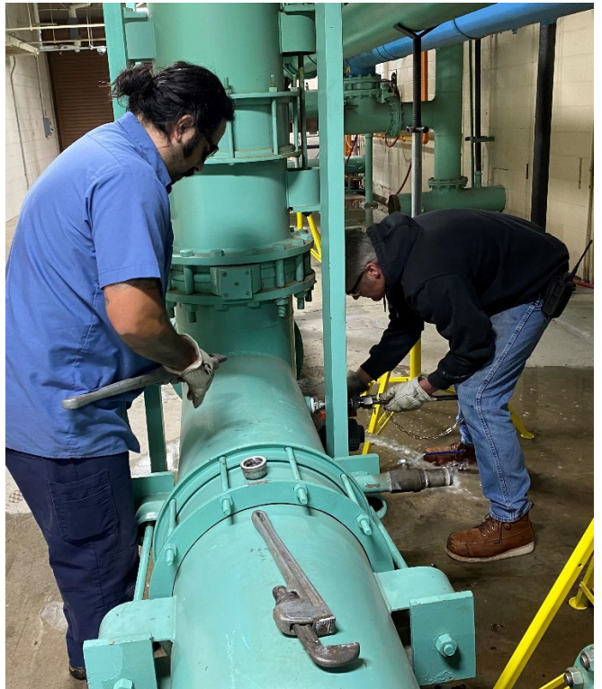
Injection Quill Installation
