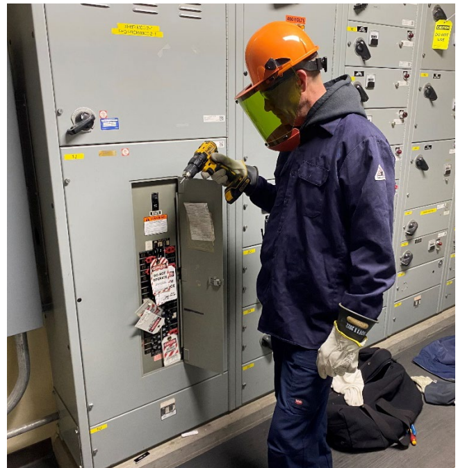
Lighting Panel Electrical Work
