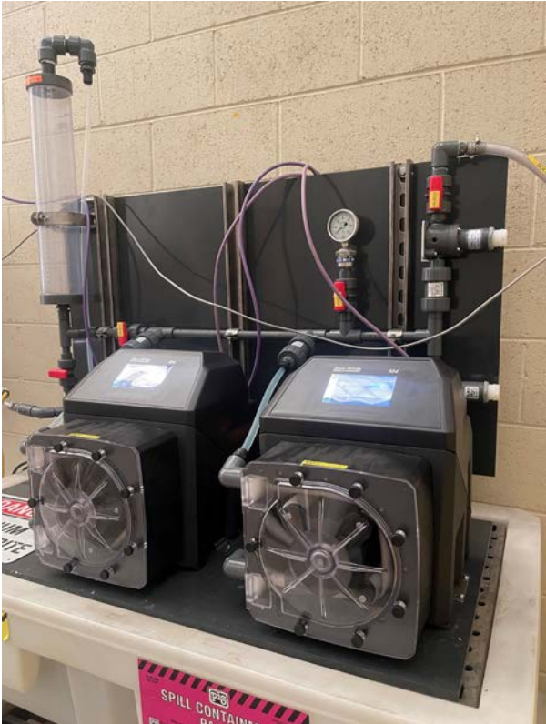
2022 Sodium Hypochlorite Disinfection Project Pump Assemblies Installed
