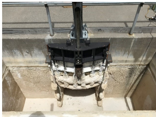
Sluice Gate
