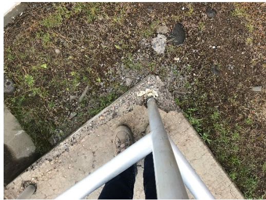
Cracking Concrete
