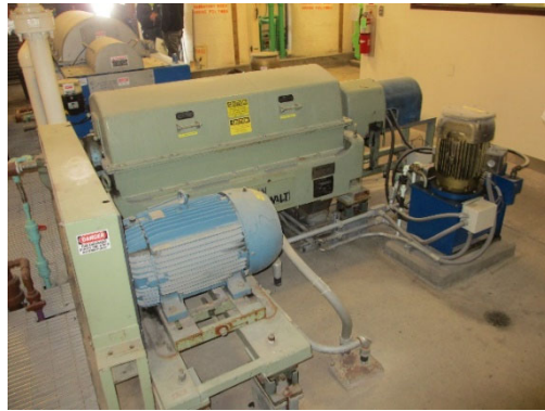
Thickening Centrifuges
