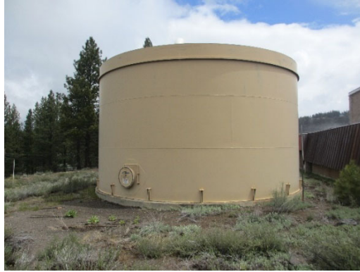
Backwash Equalization Tank
