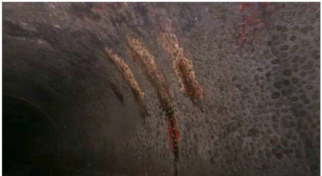
Figure 2.3 Example: Surface Reinforcement Visible (SRV) Defect
