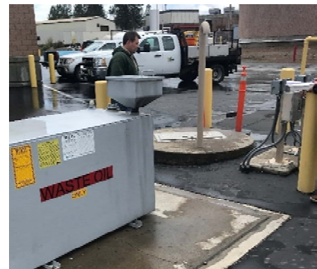
Sewage Pump Station adjacent to Facility 44
