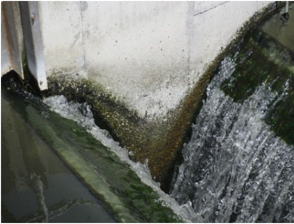
Effluent Splitter Box Concrete Aggregate
