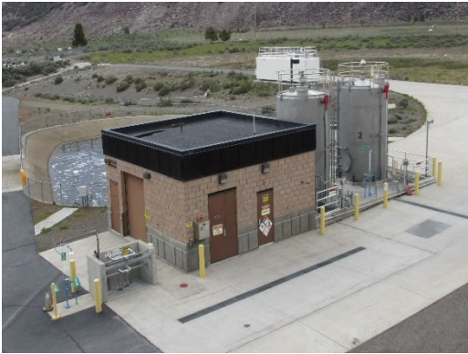
BNR Support Facility
