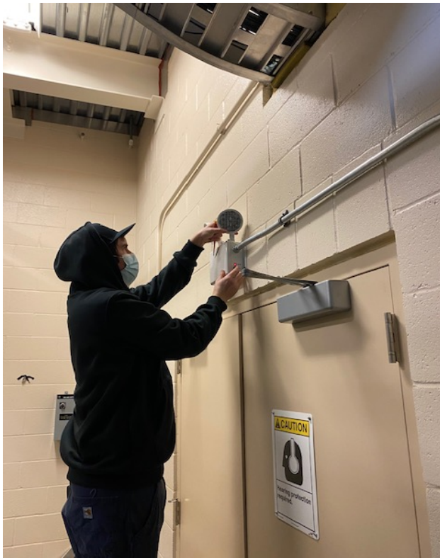
BNR Emergency Light Safety Upgrade
