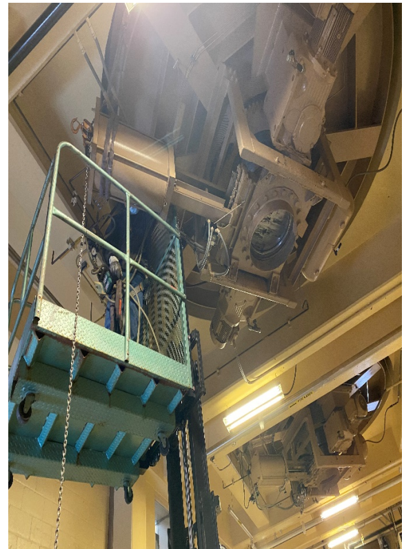
Sludge Load Out Air Cylinder Install
