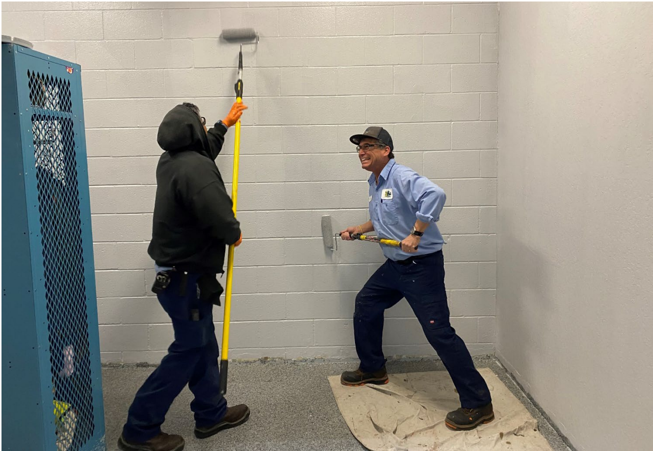
Maintenance Wet Room Painting
