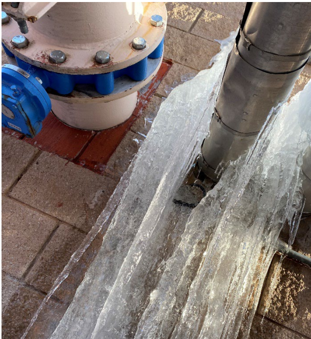
Heat Trace Repairs
