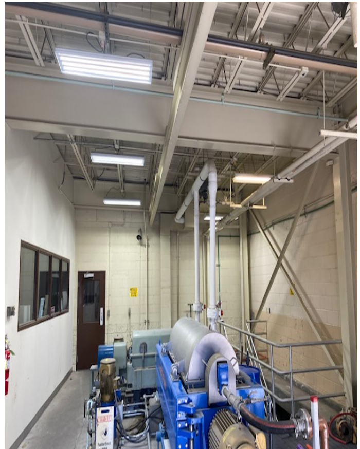
Thickening LED lighting upgrade
