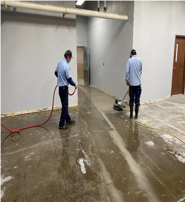
Shop floor preparation for epoxy system
