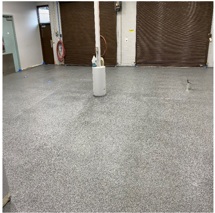
Shop floor after being coated with epoxy system
