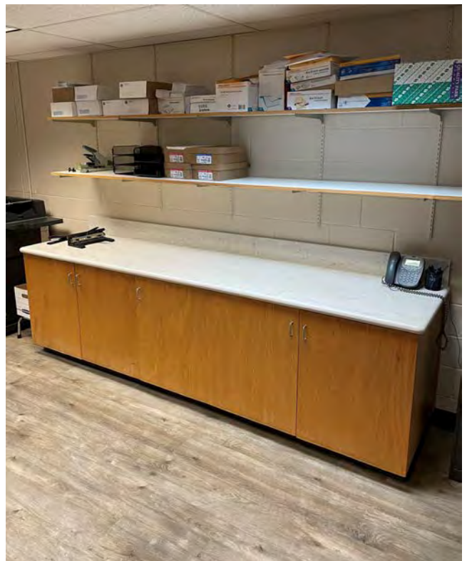
2020 Admin. Building Remodel Project Final Work Item - Counter Top After
