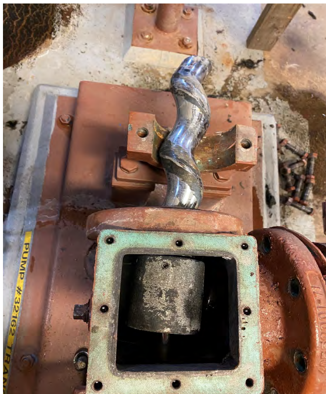
Sludge Transfer Pump Rebuild
