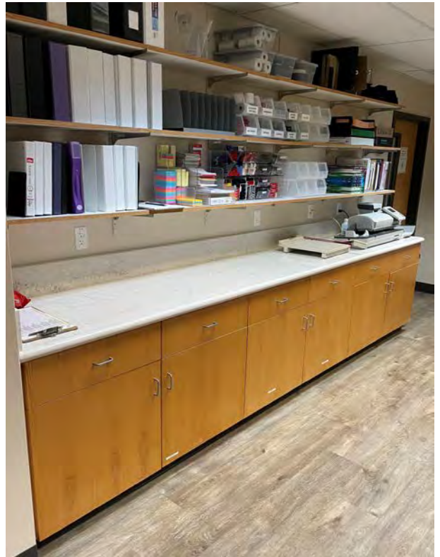
2020 Admin. Building Remodel Project Final Work Item - Counter Top After
