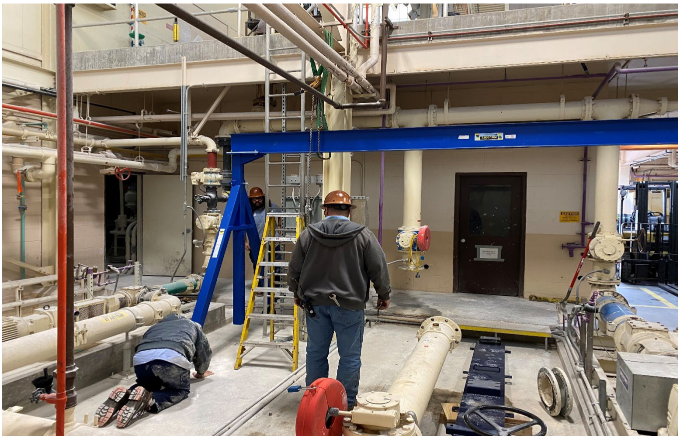
Filter Press Feed Pump Replacement
