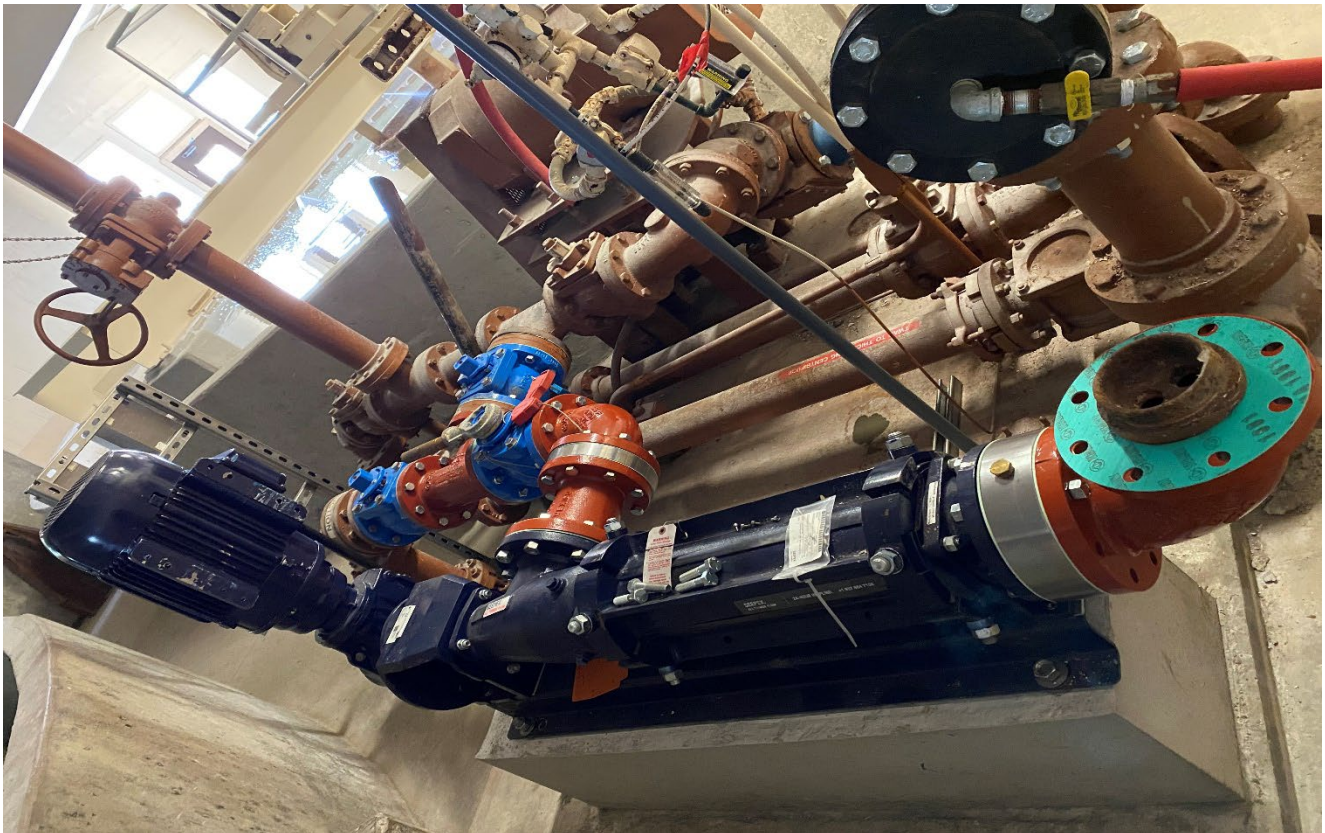
TWAS Pump Replacement
