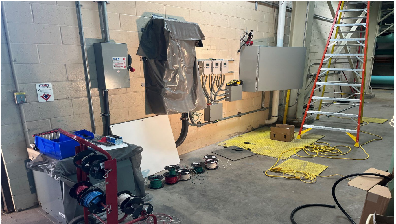
Sodium Hypochlorite Project - Electrical and Instrumentation
