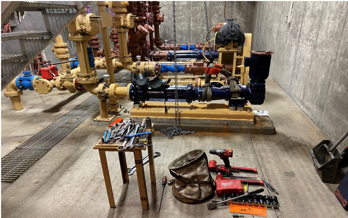
Primary Scum Pump Replacement
