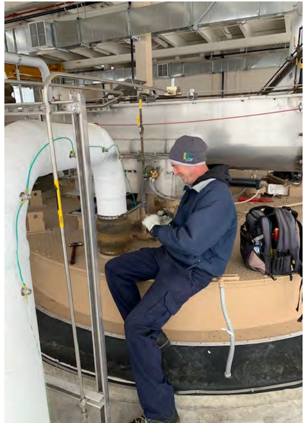
Dewatering Hopper Gate Repair
