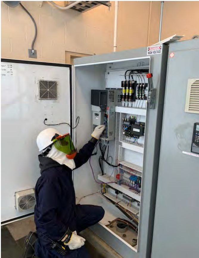
Centrifuge # 2 VFD Replacement
