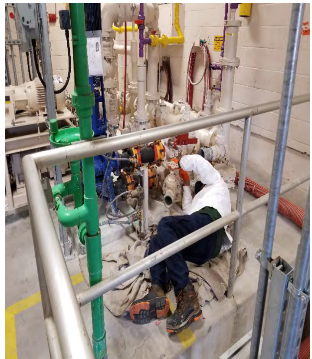
Pump Station 23 Painting Project
