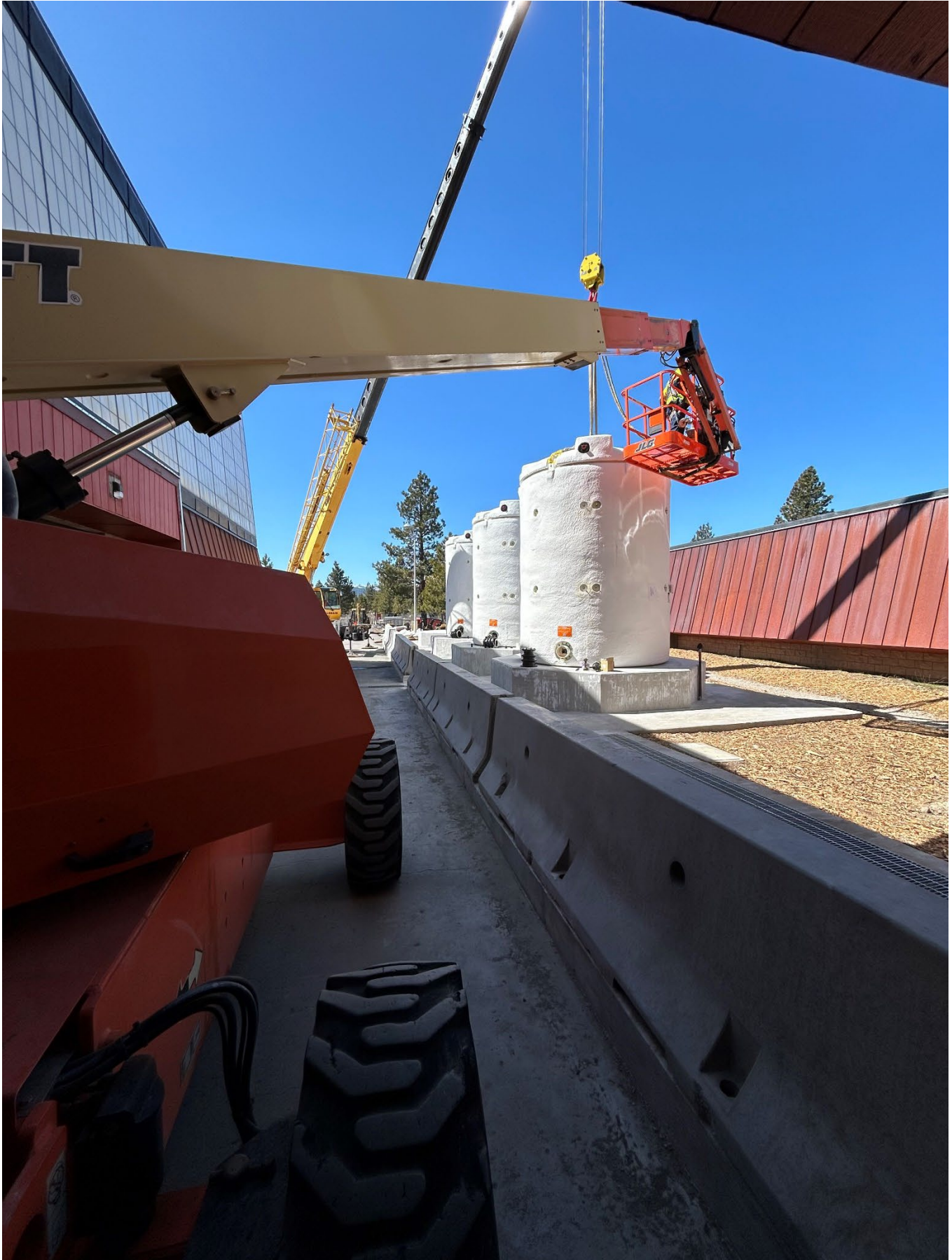
Sodium Hypochlorite Tank Installation
