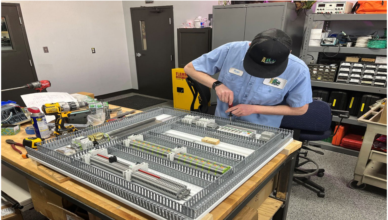
Sodium Hypochlorite Project – Remote I/O Panel
