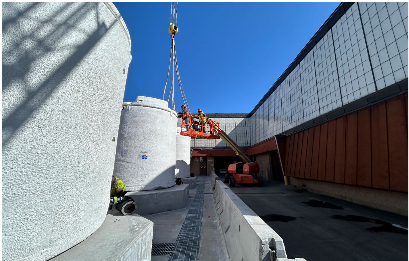
Sodium Hypochlorite Tank Installation
