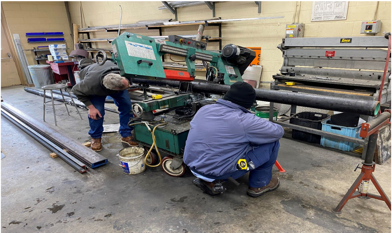
Primary Scum Pump Pipes
