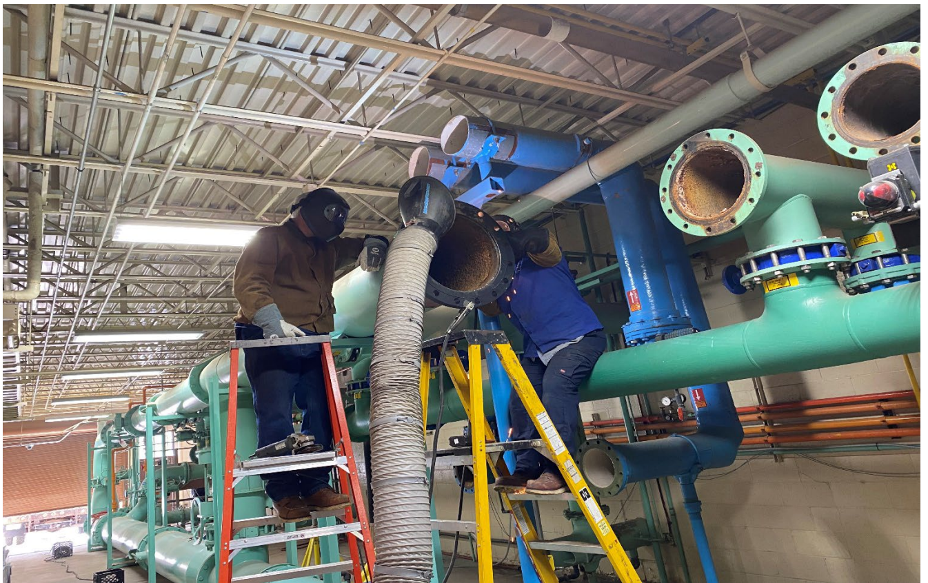
Final Effluent Spool Welding
