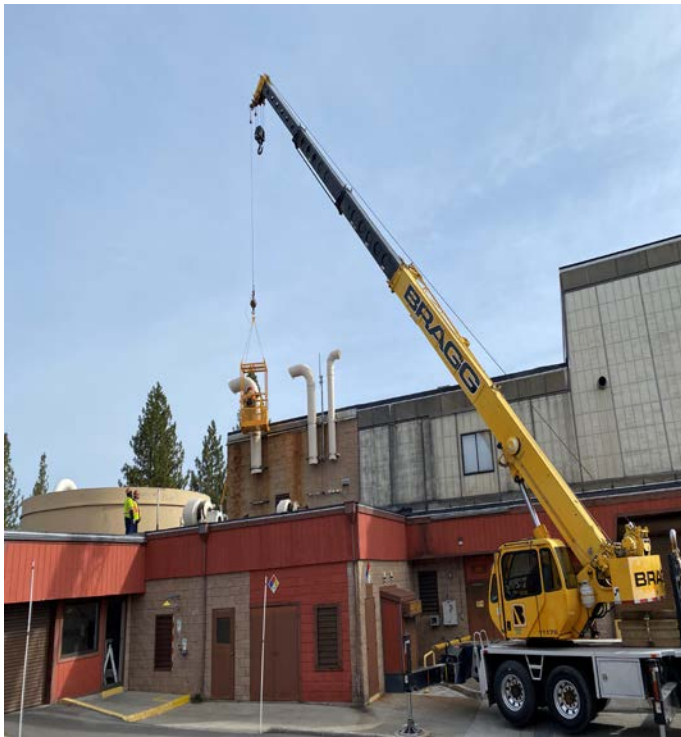
Demolition of duct 2022 Roofing Project
