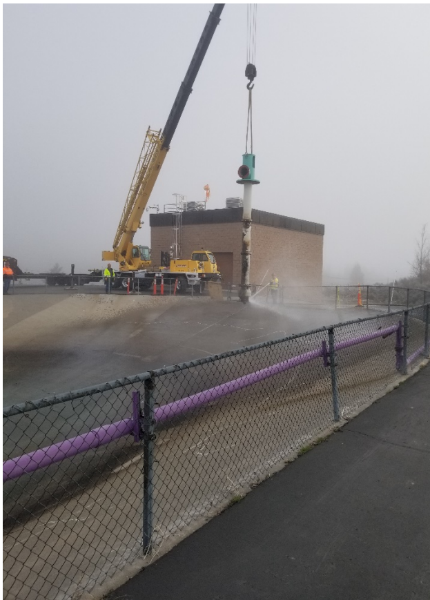
Removal of BNR influent pump #1
