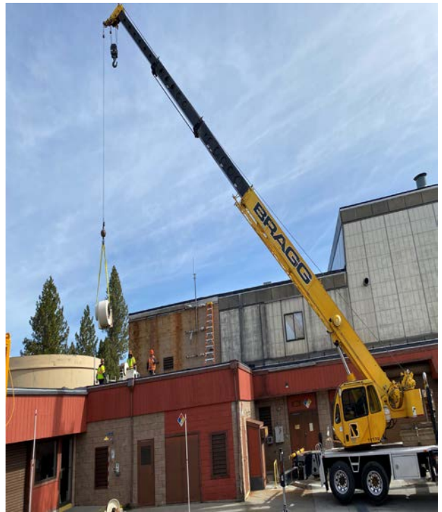
Demolition of fans for 2022 Roofing Project
