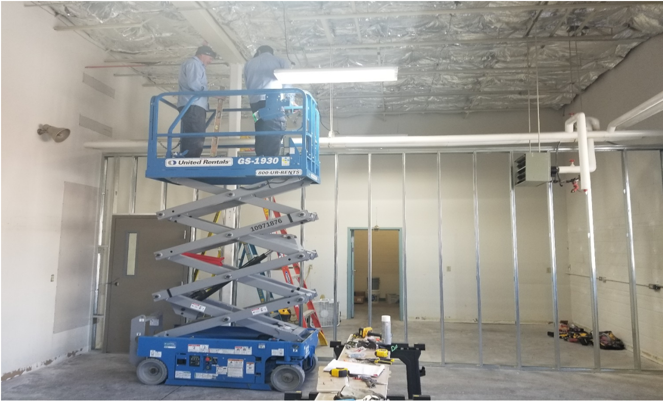
Shop relocation work
