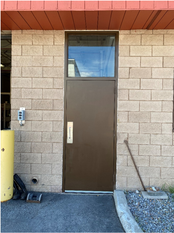
Shop door replacement
