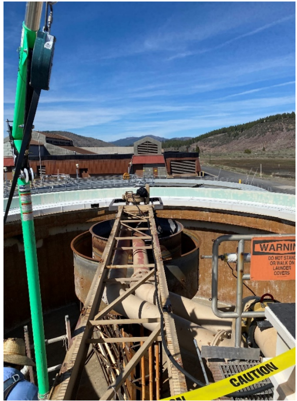
Stripper 58 teardown for coating project
