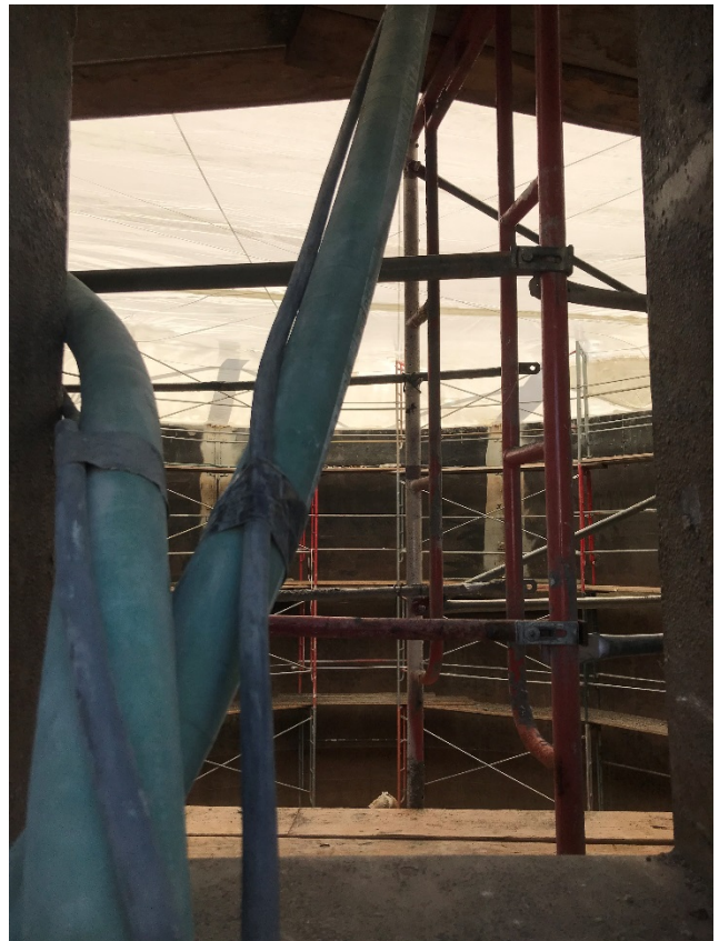
2020 Plant Painting Project – Digester 31 Interior
