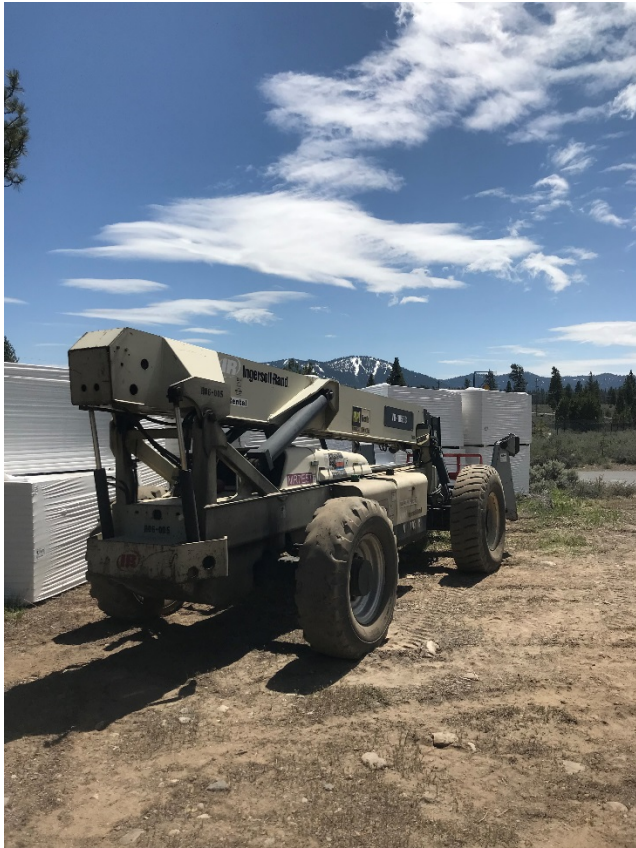
2019 Roof Repair Project – Contractor Mobilization
