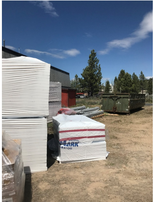
2019 Roof Repair Project – Insulation Onsite
