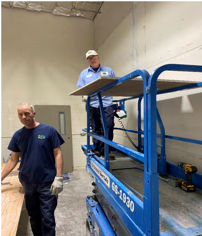
Shop relocation work
