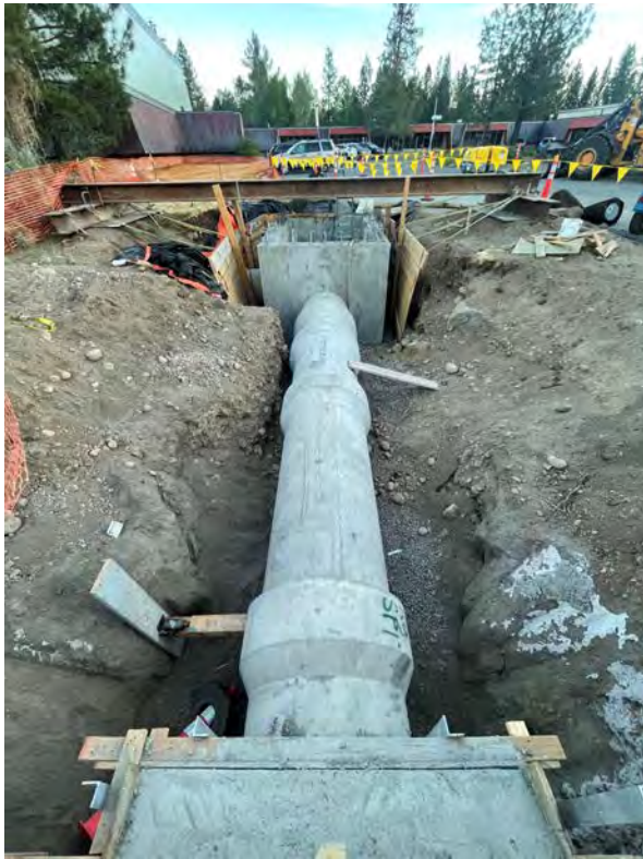
2020 Headworks Improvements Project Upstream Diversion Structure
