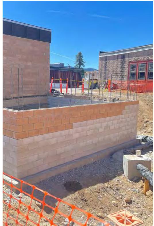
2020 Headworks Improvements Project Expansion of Headworks Building
