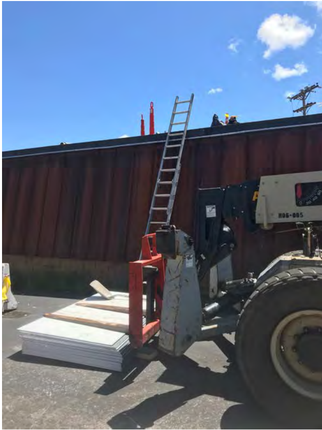
2019 Roof Repair Project – Electrical Supply Building
