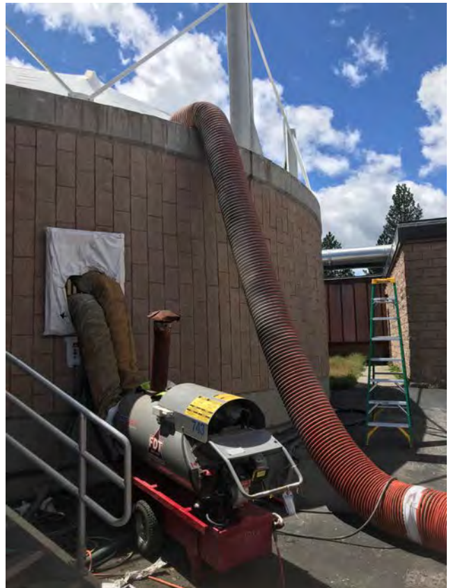
2020 Plant Painting Project – Digester 31 Painting
