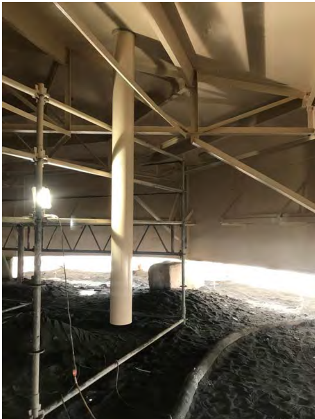
2020 Plant Painting Project –Coating Floating Cover
