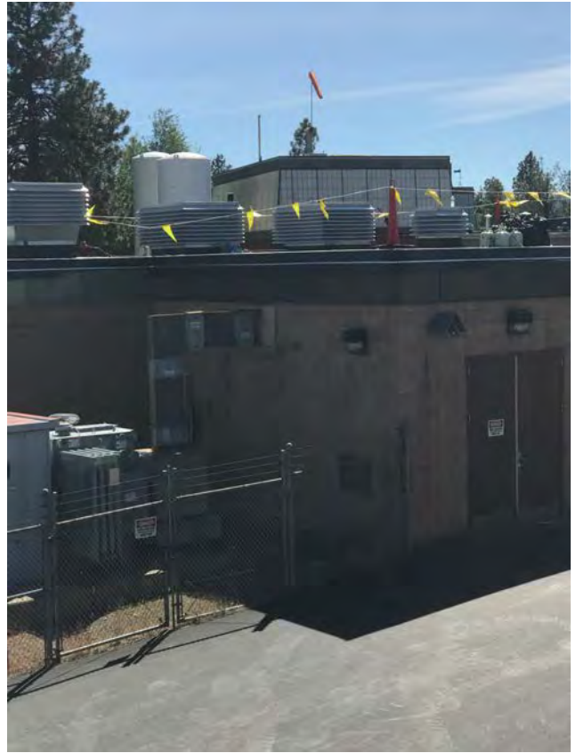
2019 Roof Repair Project – Electrical Supply Building
