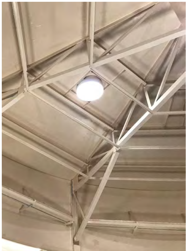
2020 Plant Painting Project – Digester 31 Cover
