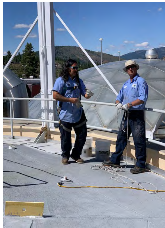
Digester 31 piping project
