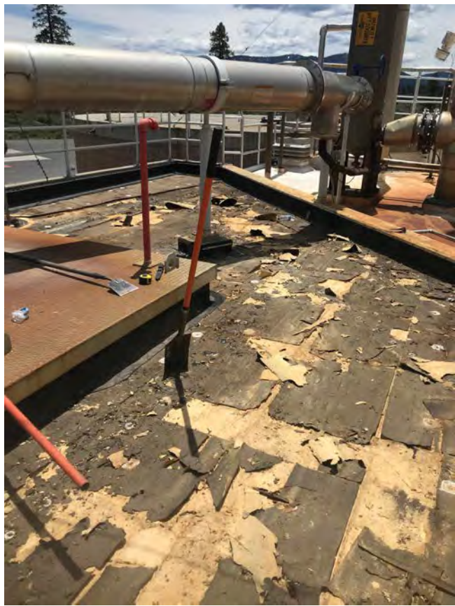
2019 Roof Repair Project – Digester Building
