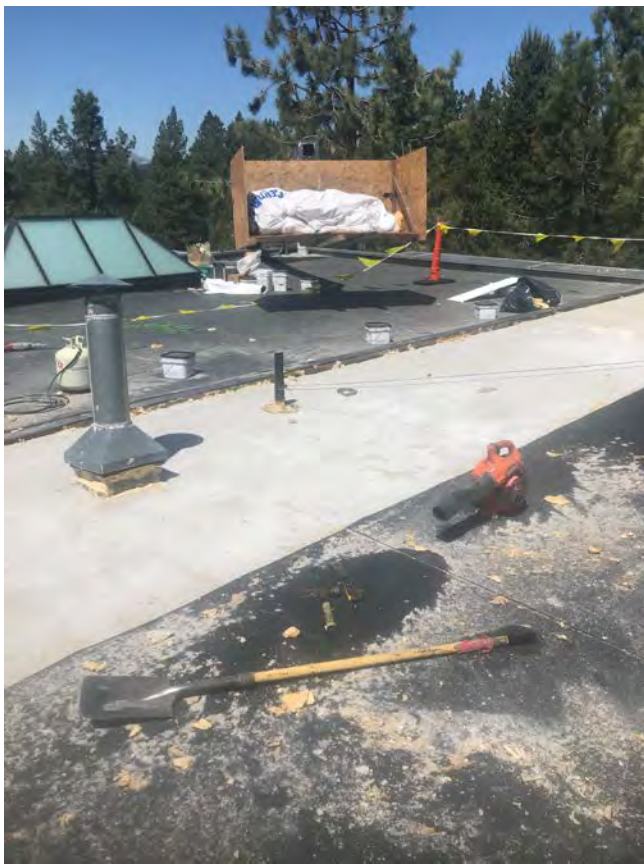
2019 Roof Repair Project – Administration Building
