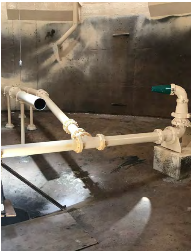
2020 Plant Painting Project – Digester 31 Interior
