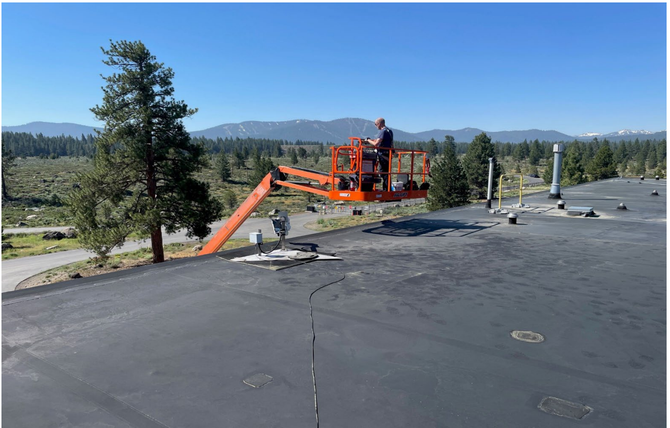
Roof Repair Project Support
