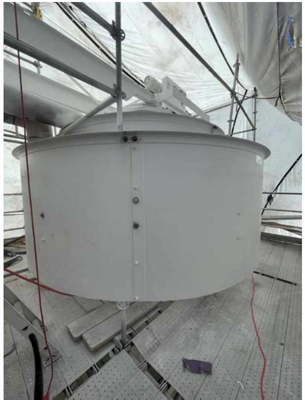
2022 Plant Coating Project Stripper Basin No. 57 – Prime Coat
