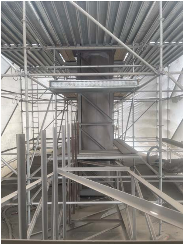
2022 Plant Coating Project Stripper Basin No. 57 – Prime Coat
