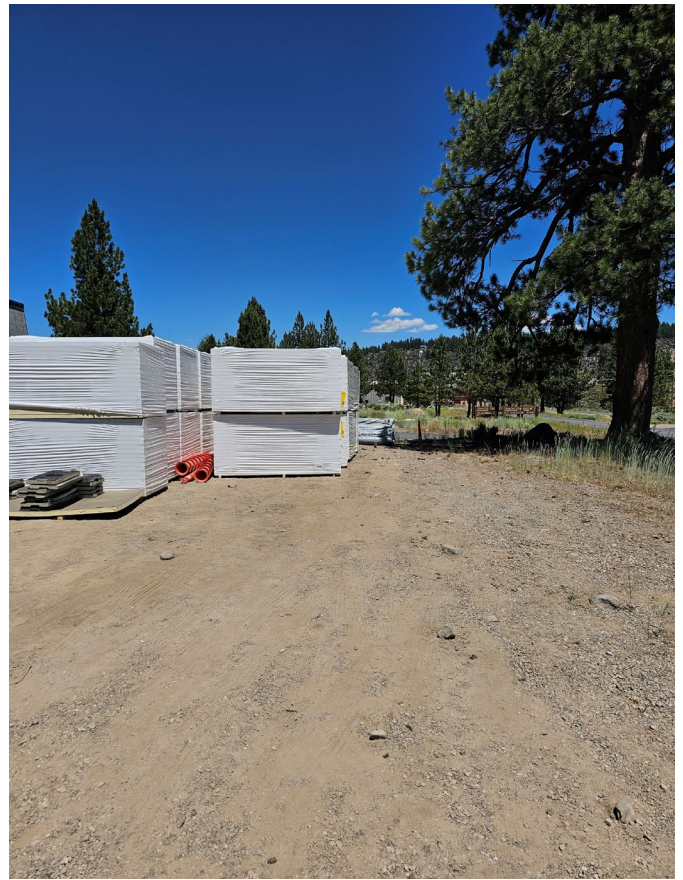
2023 Roof Repair Project Delivery of Materials
