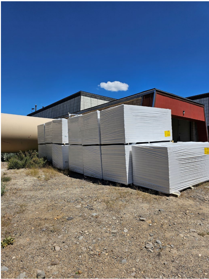
2023 Roof Repair Project Delivery of Materials
