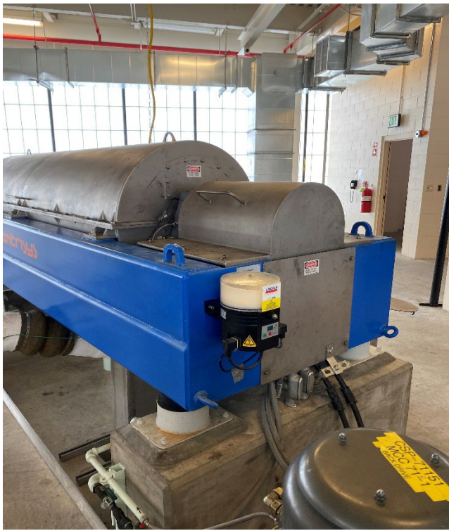
Centrifuge Auto Lube Unit Replacement
