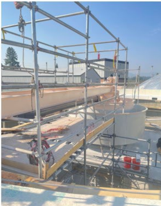
2022 Plant Coating Project Stripper Basin No. 57 – Finish Coat
