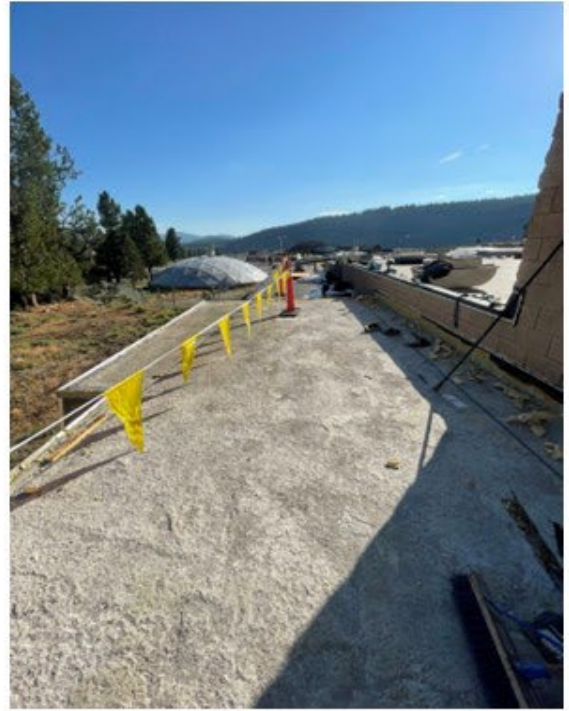
2022 Roof Repair Project Building 4 & Roof Over Corridor 6A – During Construction
