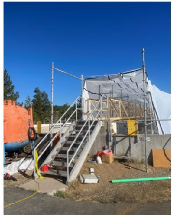
2022 Plant Coating Project Secondary Clarifier No. 2 – Installation of Dust Containment
