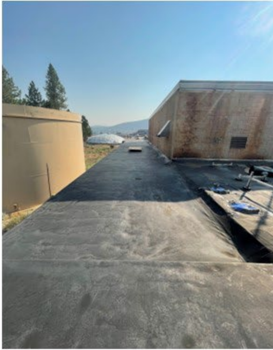
2022 Roof Repair Project Building 4 & Roof Over Corridor 6A – Pre-Construction
