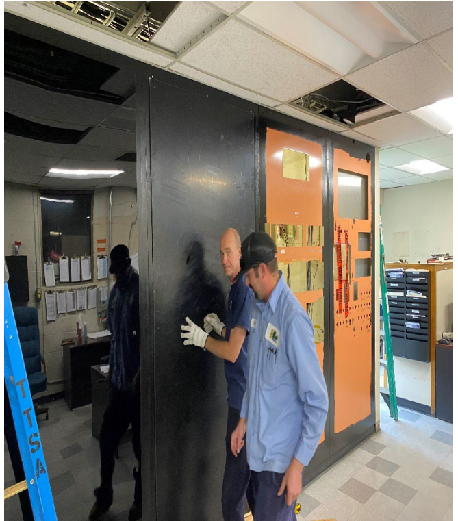
AWT Control Panel Upgrade Work
