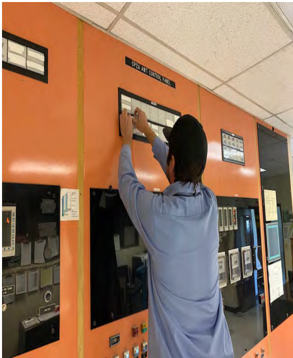
Chlorine Panel Alarm Upgrades
