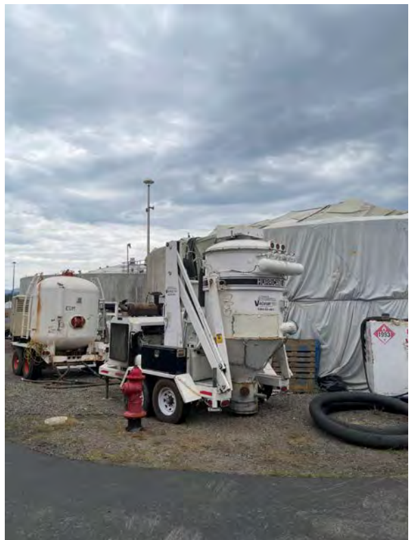
2021 Plant Painting Project Stripper Basin No. 58
