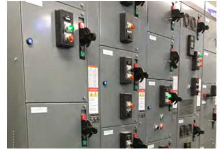
Programming and EI&C work at Big Cottonwood WTP
