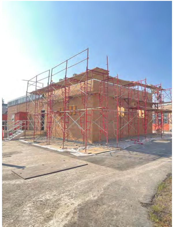
2020 Headworks Improvements Project Expansion of Headworks Building
