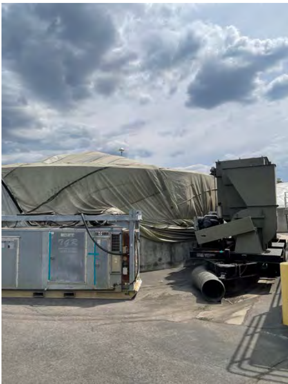
2021 Plant Painting Project Stripper Basin No. 58
