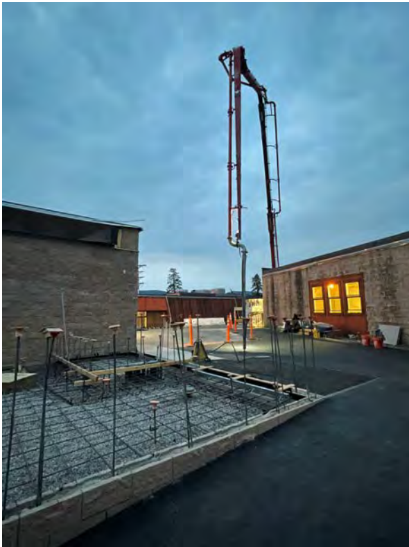
2020 Headworks Improvements Project Expansion of Headworks Building
