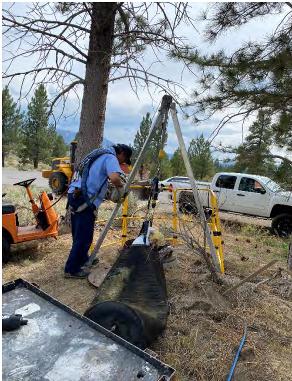
Inflatable Plug Installation
