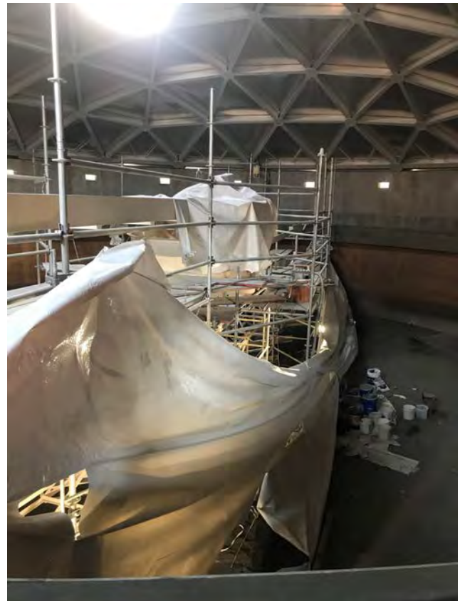
2020 Plant Painting Project – Primary Clarifier 66
