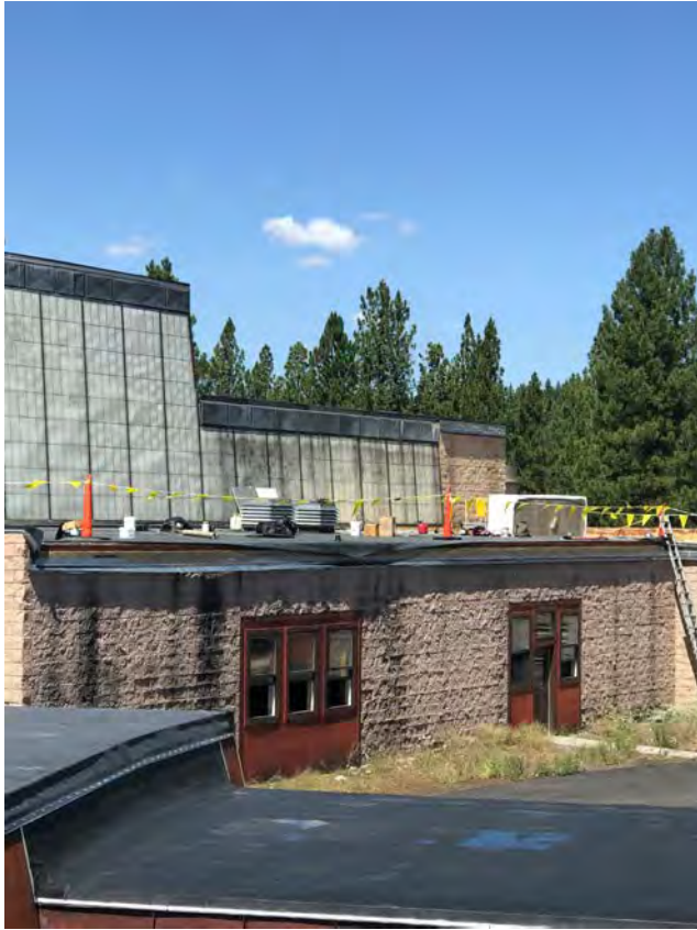
2019 Roof Repair Project – Building 4 (Thickening)
