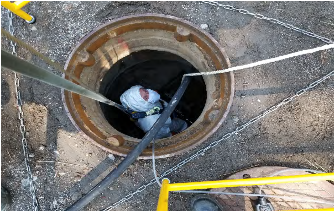
Entry into TRI MH-87 to place root cutter
