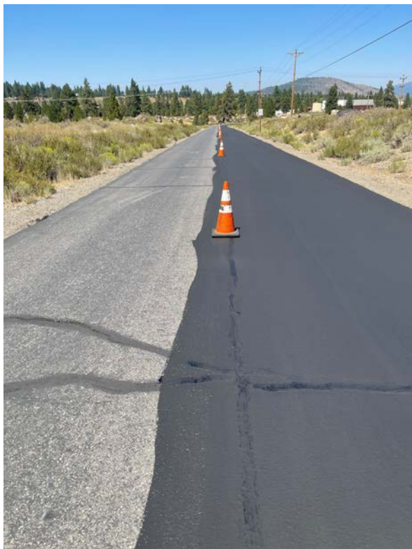
2021 Asphalt Sealing Project Access Road – In Progress
