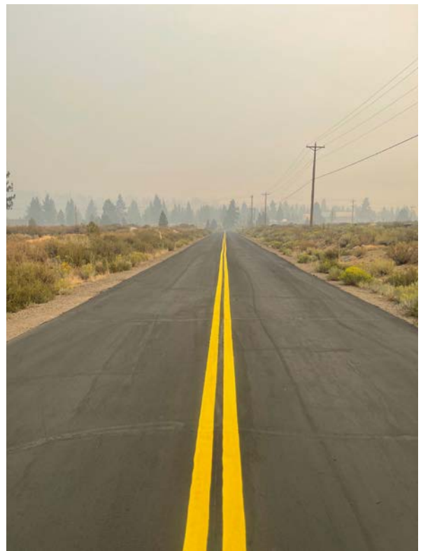
2021 Asphalt Sealing Project Access Road – After
