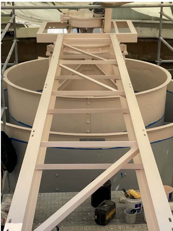
2021 Plant Painting Project Stripper Basin No. 58
