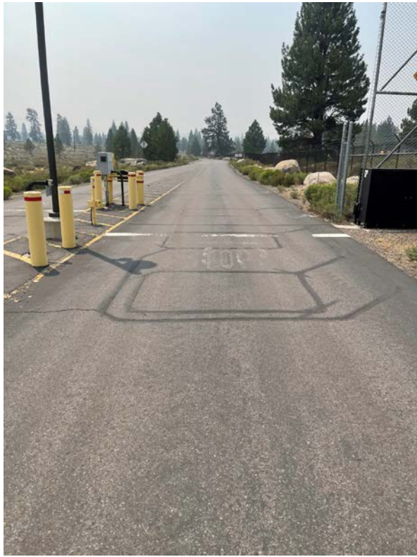
2021 Asphalt Sealing Project Front Gate - Before
