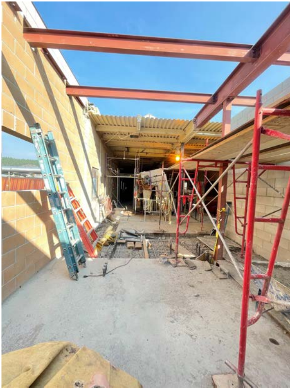
2020 Headworks Improvements Project Expansion of Headworks Building
