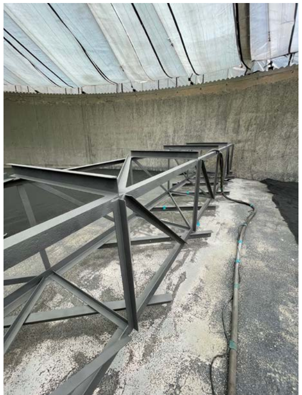
2021 Plant Painting Project Secondary Clarifier No. 2
