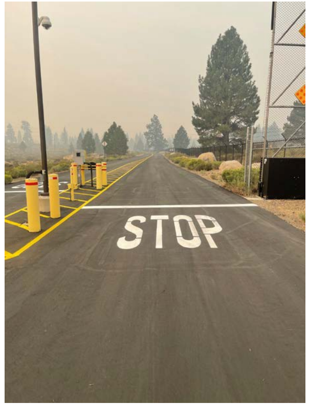
2021 Asphalt Sealing Project Front Gate - After
