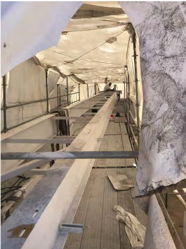
2020 Plant Painting Project – Secondary Clarifier 54
