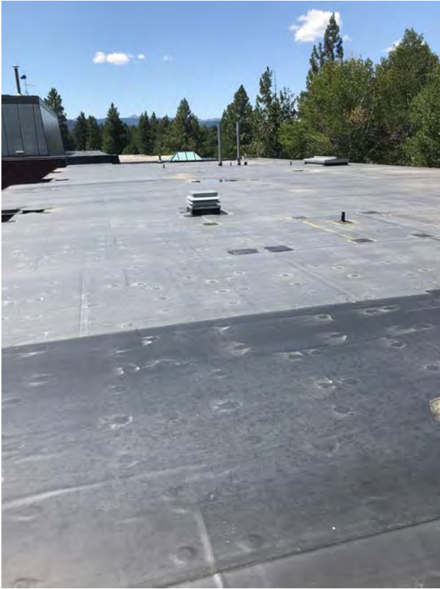
2019 Roof Repair Project – Building 1 (Administration)
