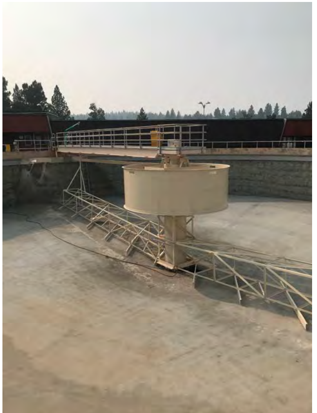
2020 Plant Painting Project – Secondary Clarifier 54
