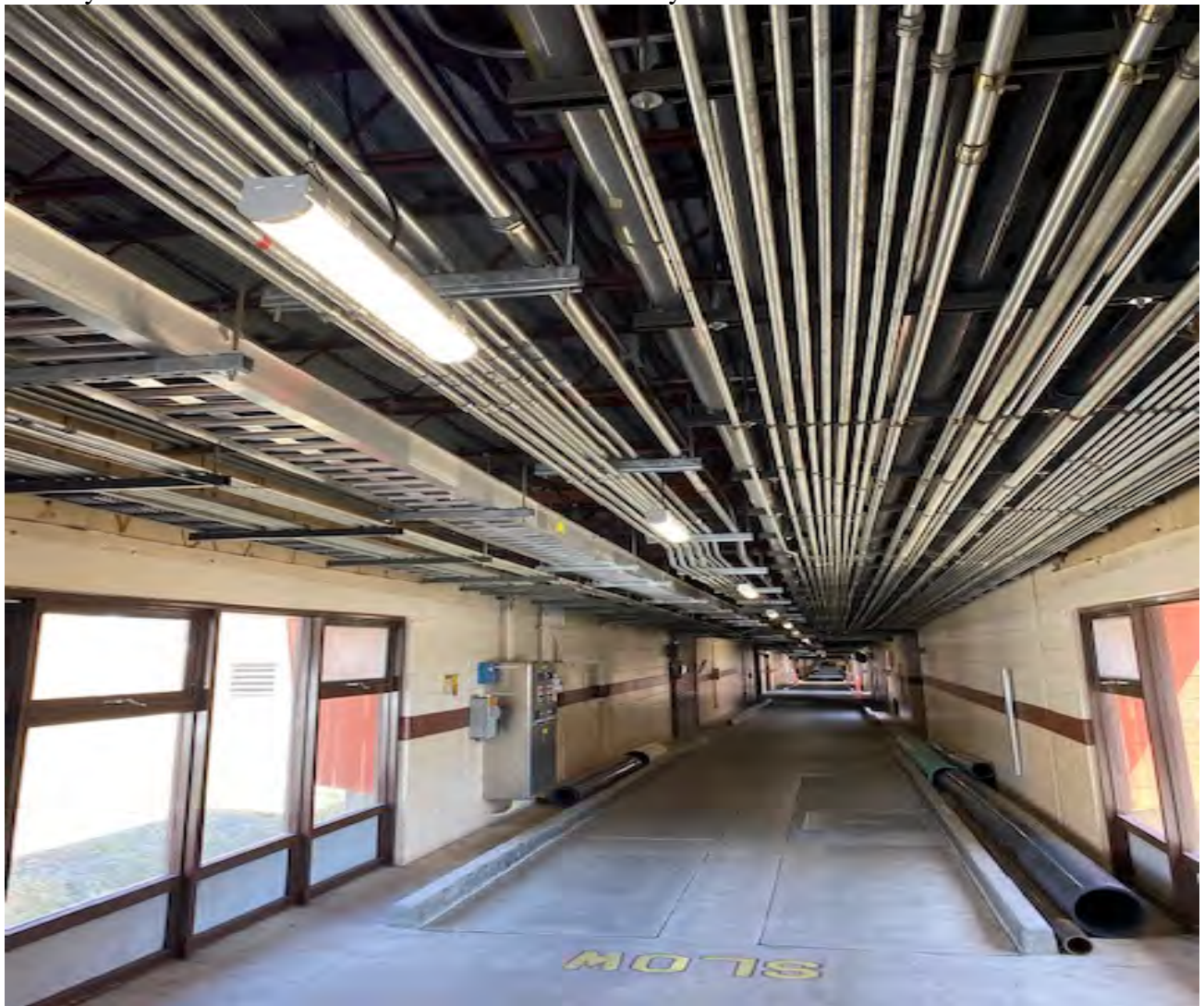
Corridor Lighting Project
