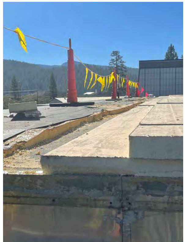
2022 Roof Repair Project Building 3 – Construction
