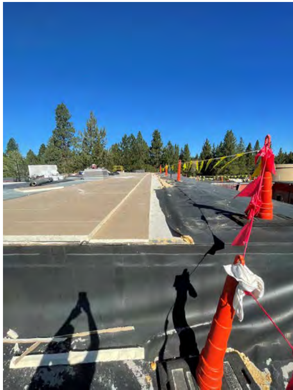
2022 Roof Repair Project Building 3 – Construction
