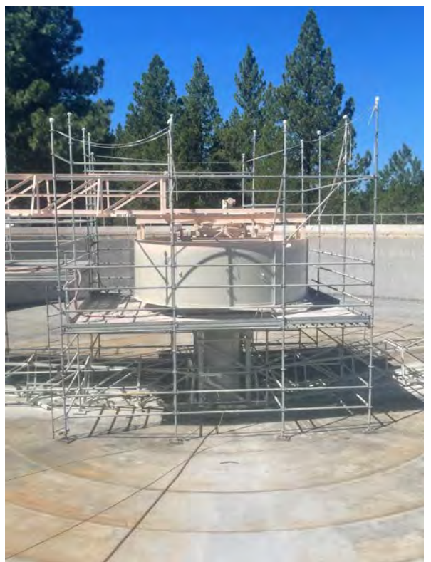
2022 Plant Coating Project Secondary Clarifier No.2 – Finish Coat
