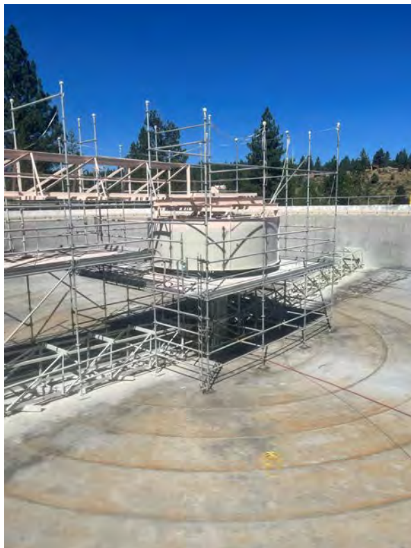
2022 Plant Coating Project Secondary Clarifier No.2 – Finish Coat
