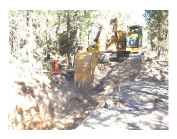
Photo 7 – Exposing the 24" DIP Section
