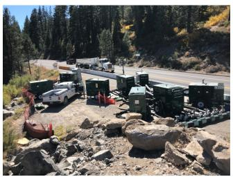
Photo 2 - Bypass Pump Station
