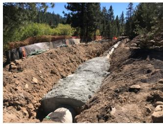
Photo 4 – Concrete Encasement Under Swale
