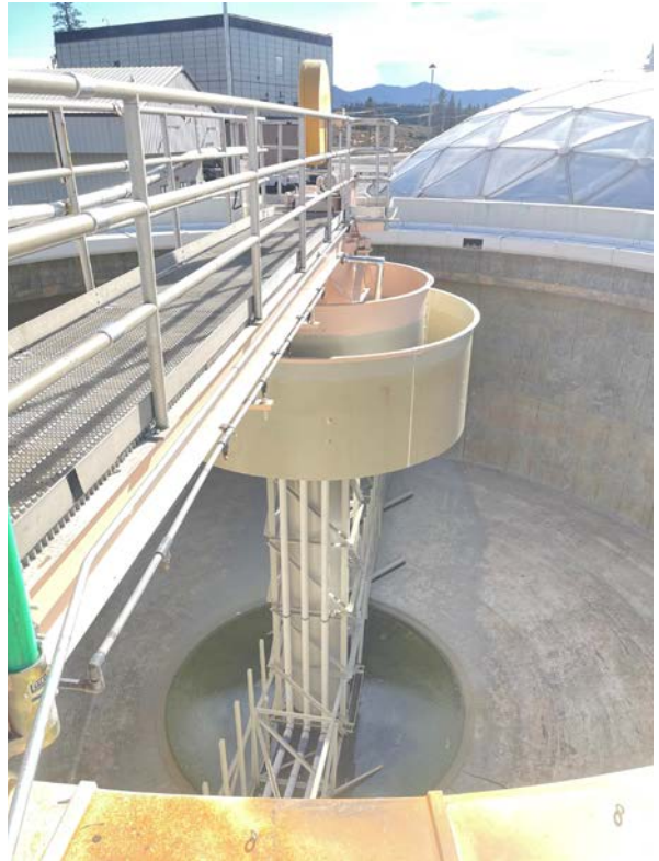
2022 Plant Coating Project Stripper Basin 57
