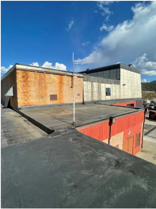
2022 Roof Repair Project Building 4 & Corridor 6A
