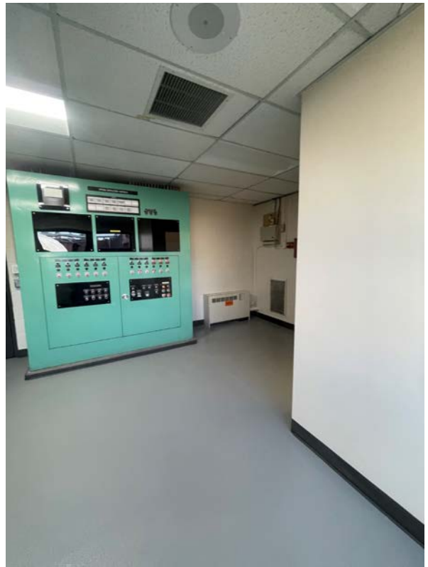
2022 Control Room Upgrades Project Building 13
