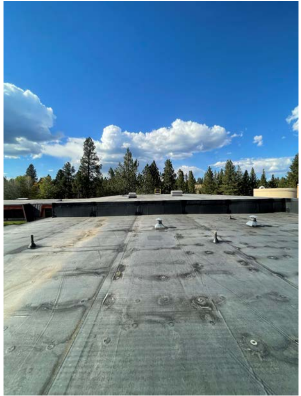
2022 Roof Repair Project Building 3
