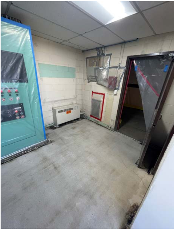
2022 Control Room Upgrades Project Building 13
