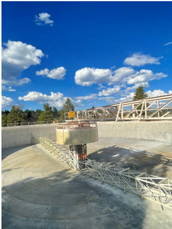
2022 Plant Coating Project Secondary Clarifier 1
