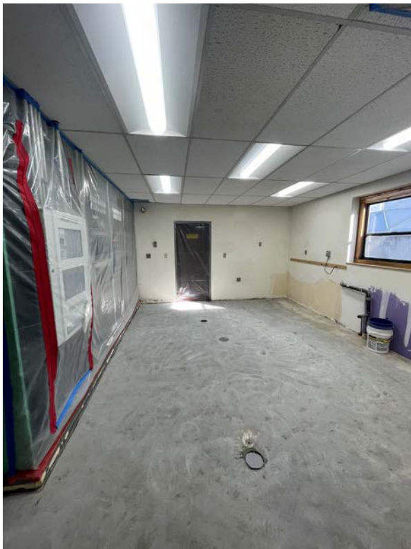
2022 Control Room Upgrades Project Building 53
