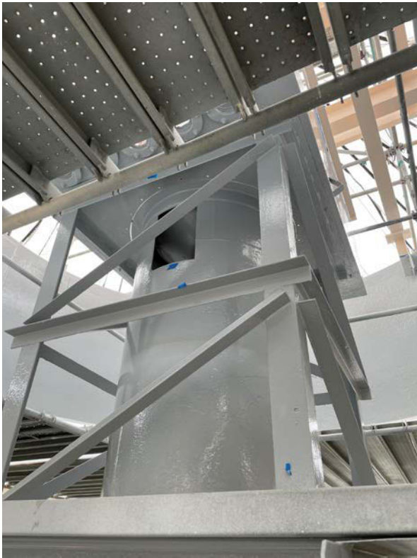
2021 Plant Painting Project Secondary Clarifier No. 2 – In Progress
