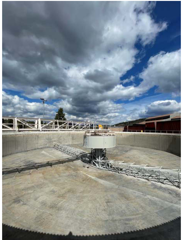
2021 Plant Painting Project Secondary Clarifier No. 2 - Complete
