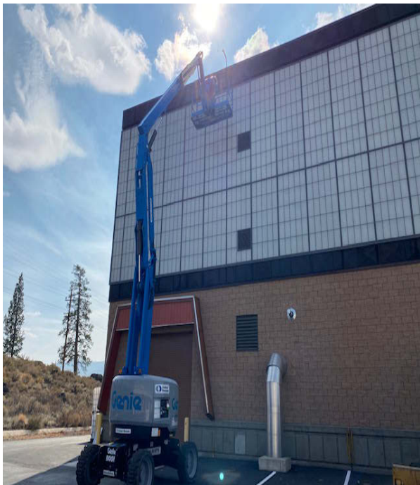
Security camera mount installation
