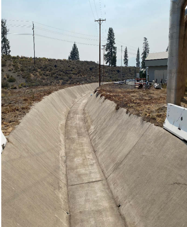
Storm channel cleanup post masitication
