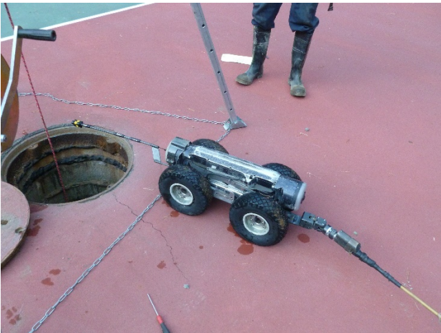
Photo 2- Digital Scanning of Sewer Lines
