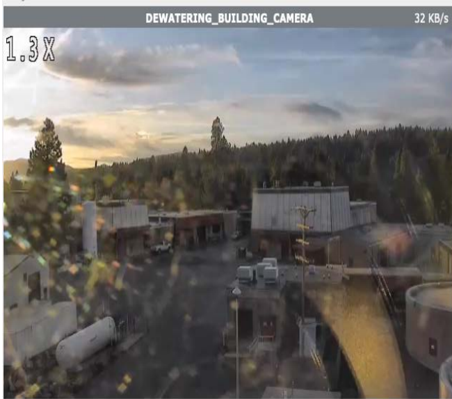
Dewatering Building Camera View
