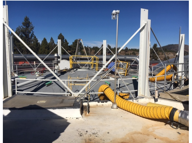
Digester Cleaning – View of Digester #31
