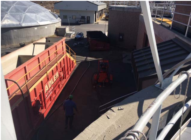
Digester Cleaning – View of Weir Tank, Filter Box & Pump
