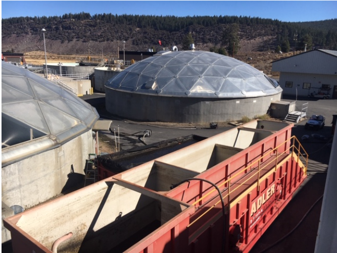
Digester Cleaning – View of Weir Tank
