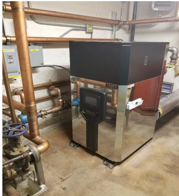
Camus Hydronic Heating Boiler
