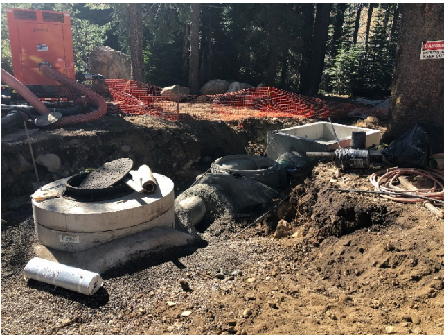
Photo 3- SVPSD Truckee River Siphon Replacement Project
