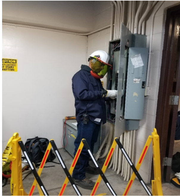
Digester PLC Power Repair
