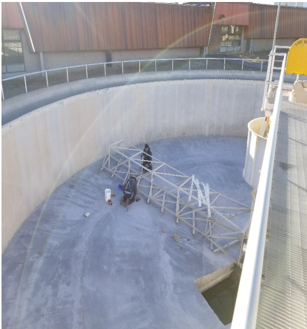
Chemical Clarifier No. 2 Wiper Installation
