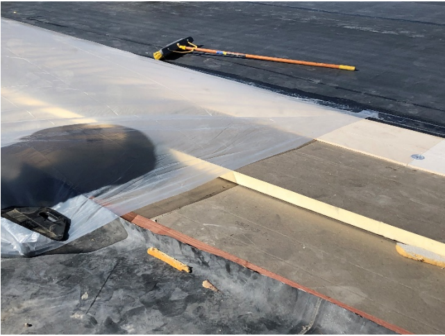
Photo 1- 2019 Roof Repair Project
