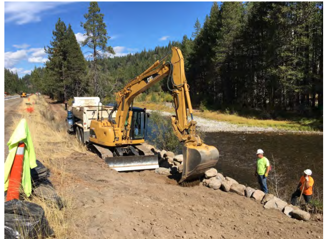
Photo 4 – Slope Restoration at “Pinch Point”
