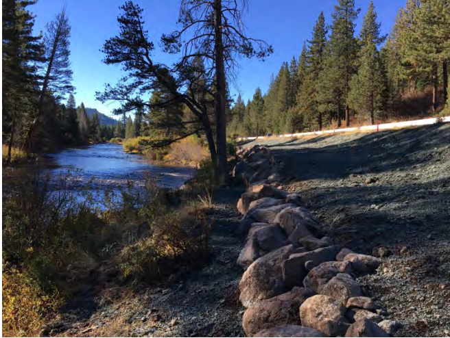
Photo 5 – Restored Slope at “Pinch Point”
