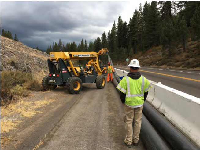
Photo 3 – Removing the Bypass Pipes
