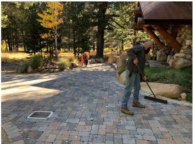
Photo 8 – Final Cleaning Of Paving Stones
