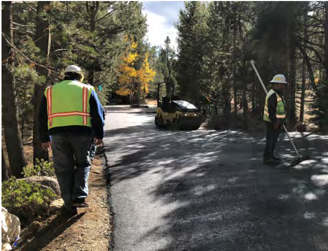
Photo 7 – Repaving the Private Driveway
