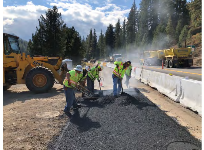
Photo 6 – Patching SR 89 Northbound Shoulder
