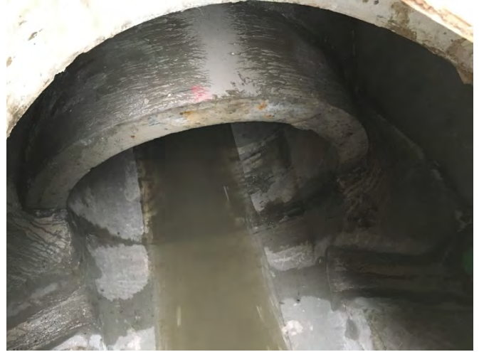
Photo 2 – Sewage Flow Restored in New Pipe
