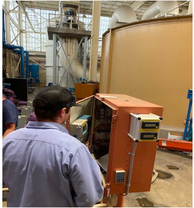
2 Water Level Device Replacment
