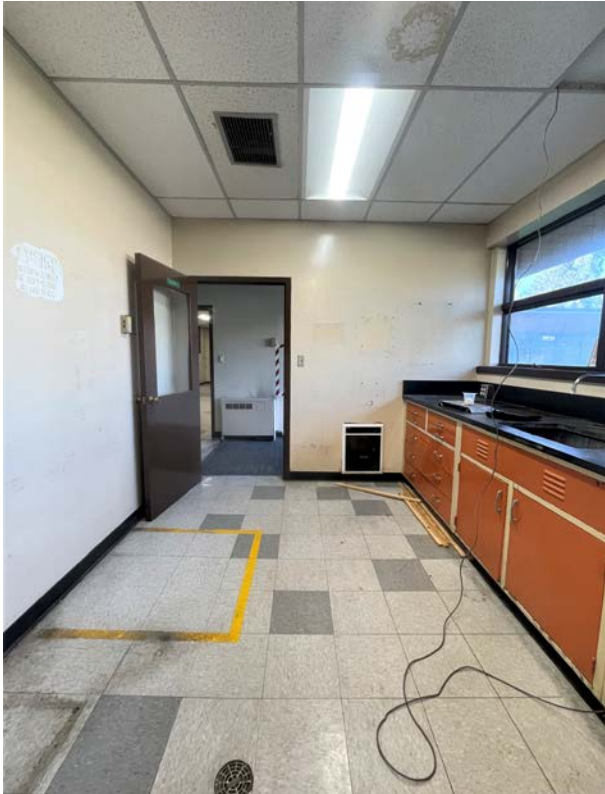
2022 Control Room Upgrades Project AWT Lab Pre-Construction
