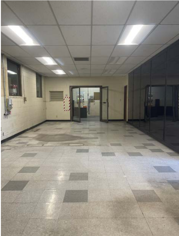
2022 Control Room Upgrades Project AWT Control Room Pre-Construction
