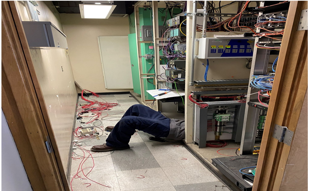
C&CT Panel Work
