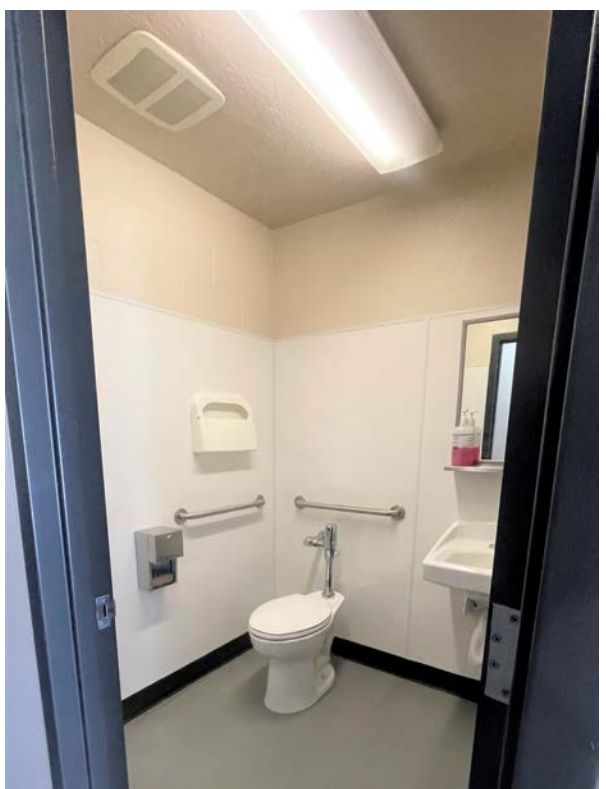
2022 Control Room Upgrades Project AWT Control Room Restroom Post-Construction
