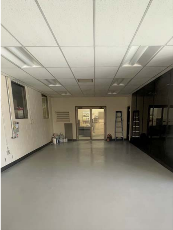
2022 Control Room Upgrades Project AWT Control Room Post-Construction
