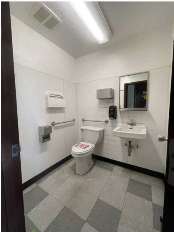
2022 Control Room Upgrades Project AWT Control Room Restroom Pre-Construction
