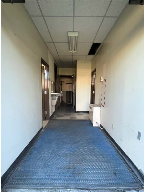
2022 Control Room Upgrades Project AWT Control Room Entryway Pre-Construction
