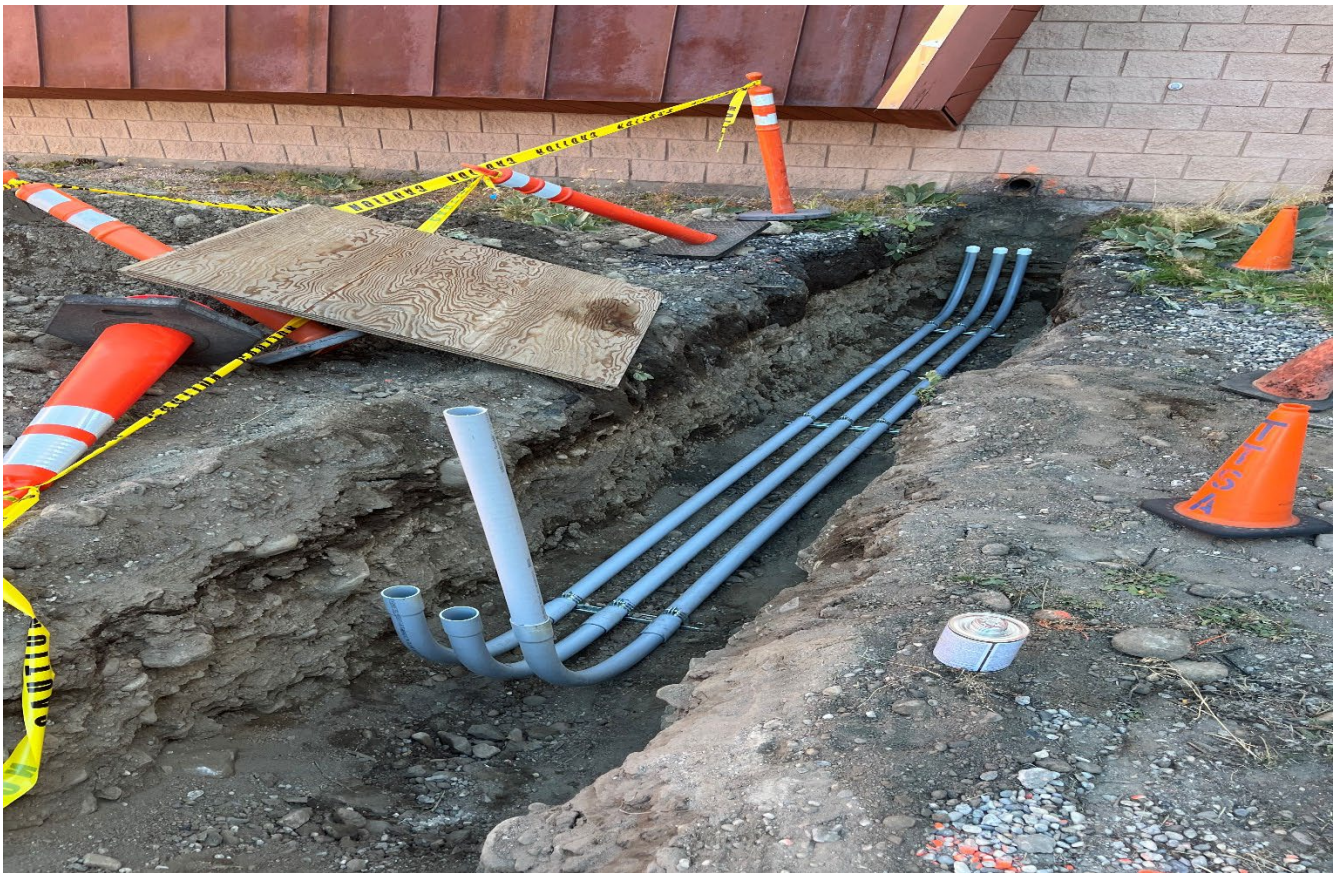
Sodium Hypochlorite Electrical Trench
