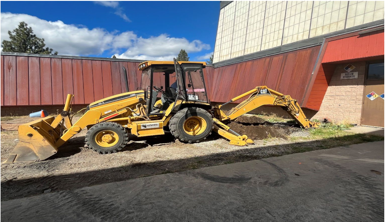
Sodium Hypochlorite Electrical Trench
