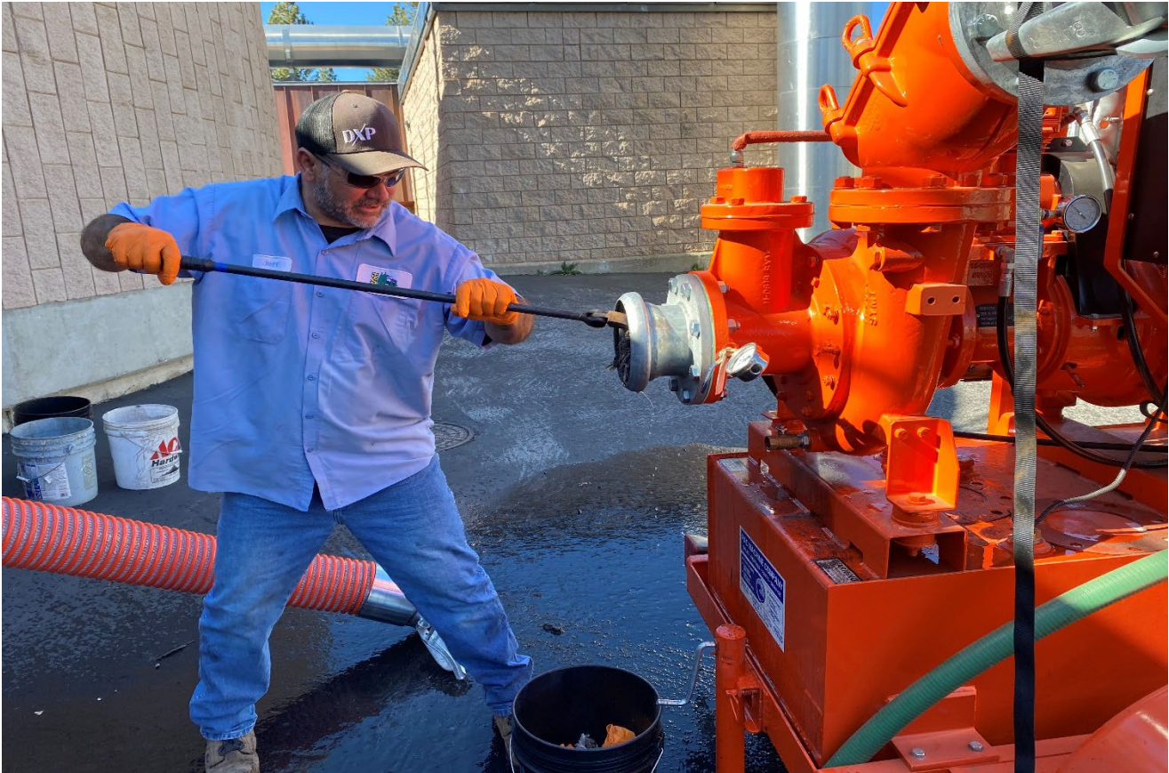
Digester Cleaning Project
