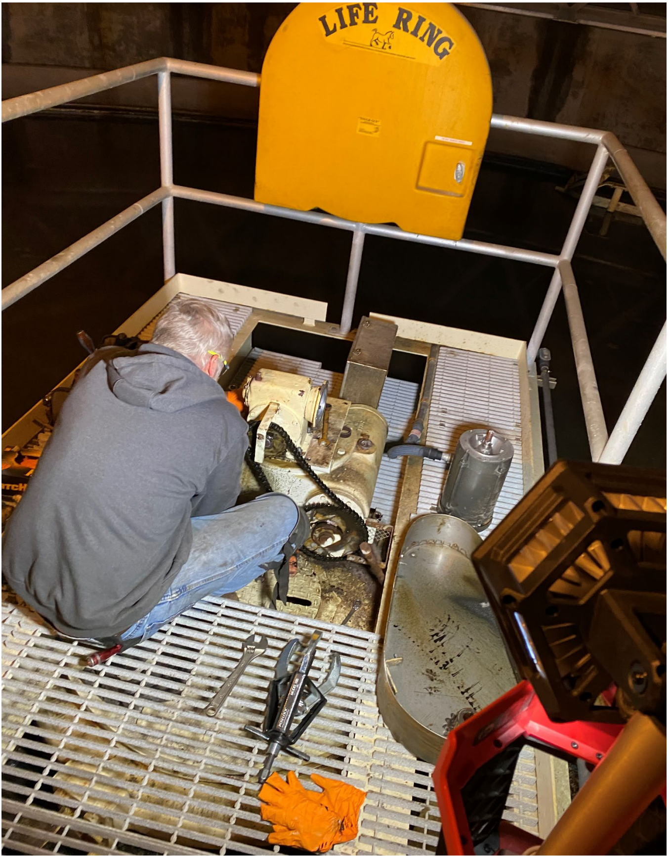
Primary #1 Gearbox Rebuild
