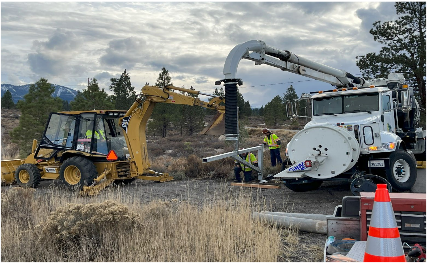
Property Gate Installation
