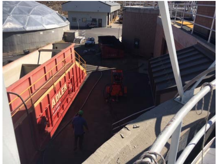
Digester Cleaning Project
