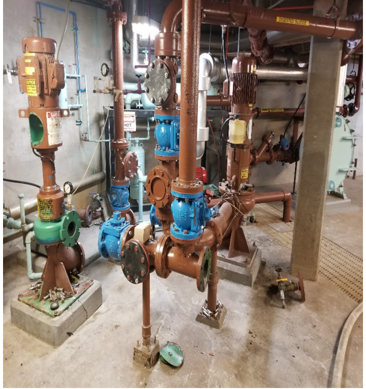
Digester Valve Replacement
