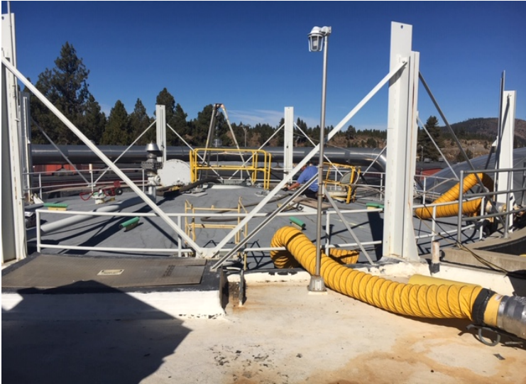
Digester Cleaning Project
