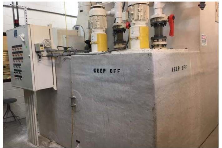
Chlorine Scrubber Tank Repair
