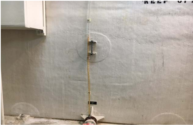
Chlorine Scrubber Tank Repair
