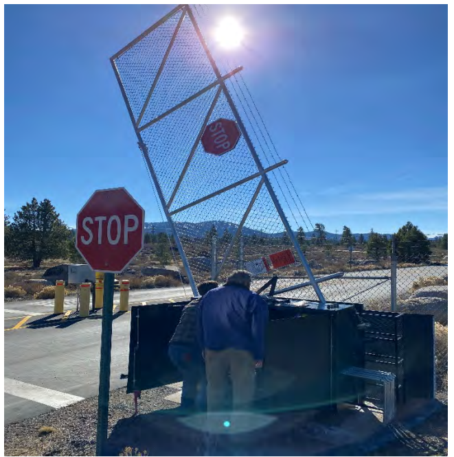
Exit Gate Replacement
