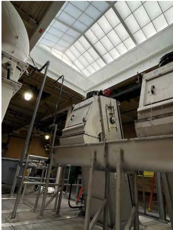
2020 Headworks Improvements Project Interior Installation Nearing Completion
