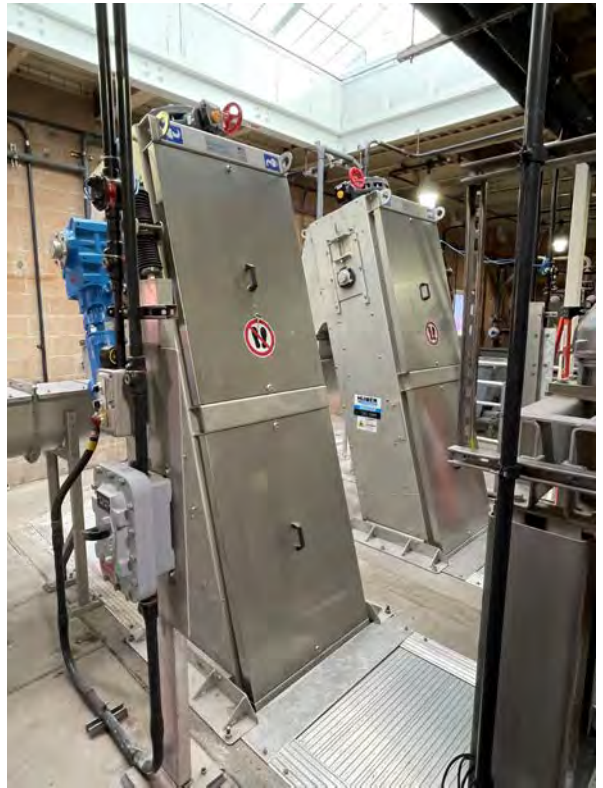
2020 Headworks Improvements Project Interior Installation Nearing Completion
