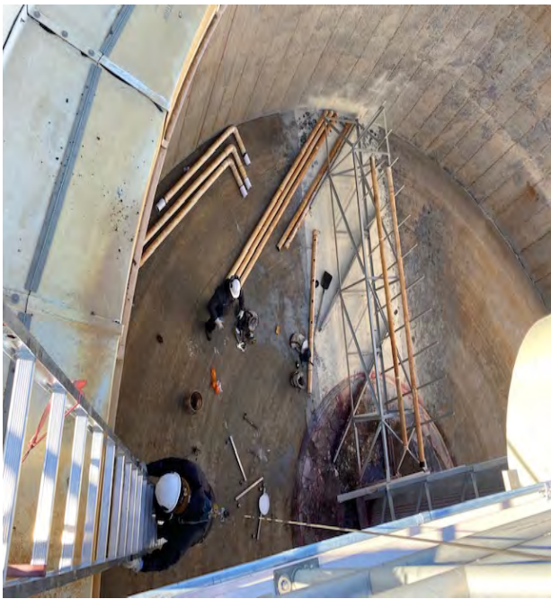
Stripper #58 Coating Project
