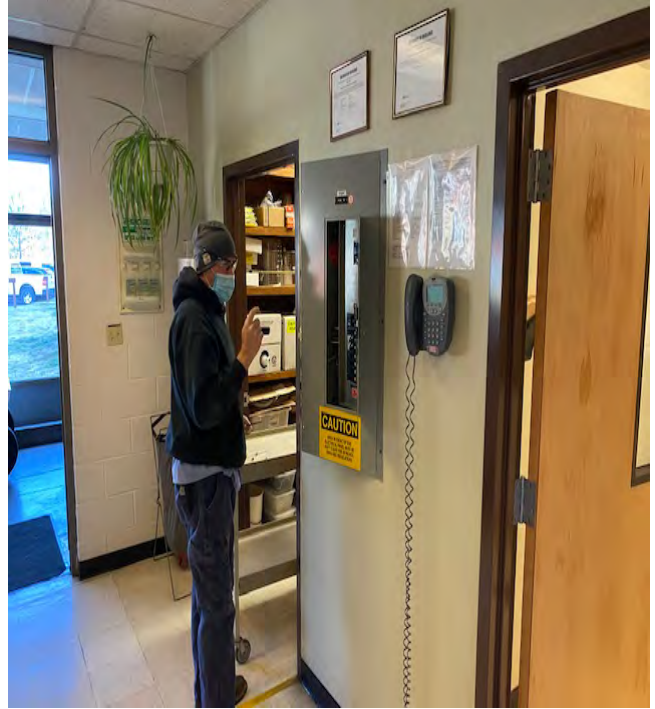
Laboratory Breaker Replacement
