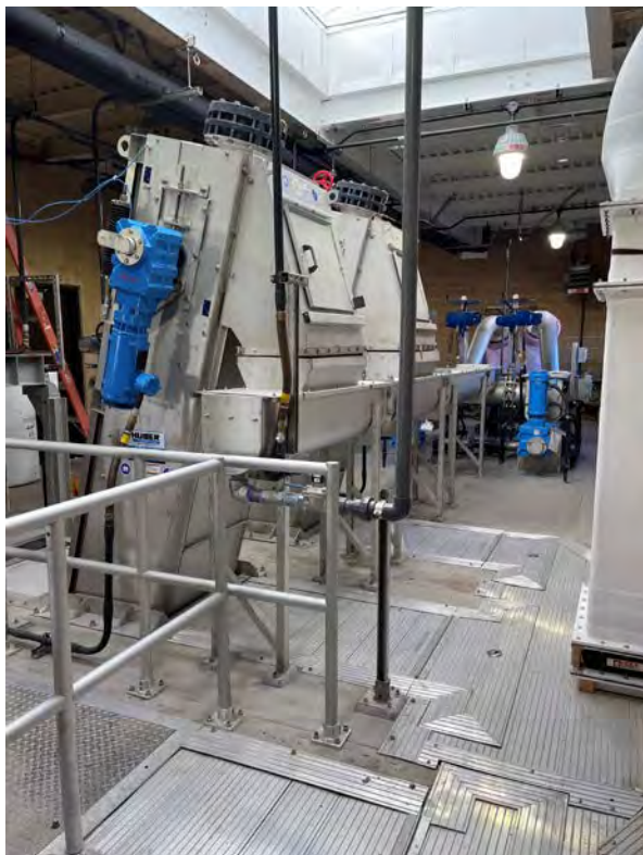
2020 Headworks Improvements Project Interior Installation Nearing Completion
