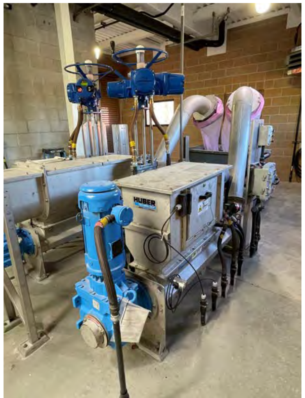
2020 Headworks Improvements Project Interior Installation Nearing Completion
