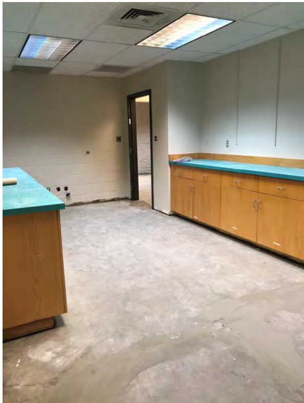
2020 Administration Building Remodel Project
