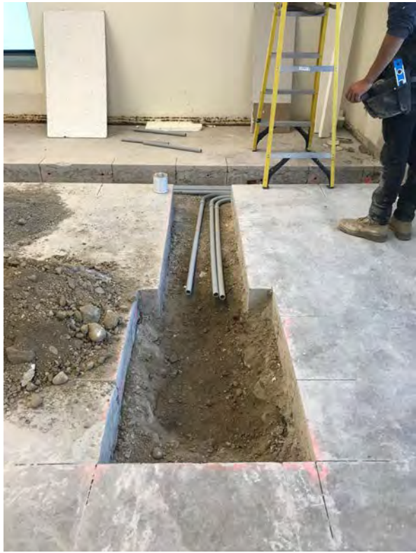
2020 Administration Building Remodel Project
