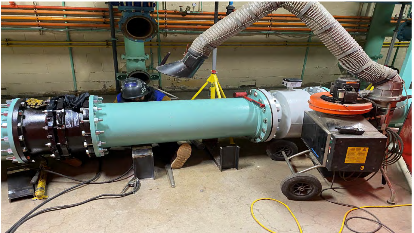
Final Effluent Flow Meter Installation
