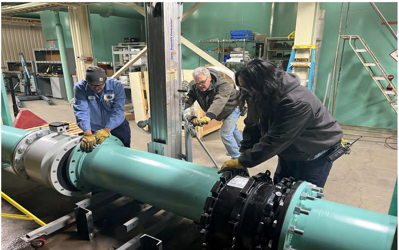
Final Effluent Flow Meter Installation
