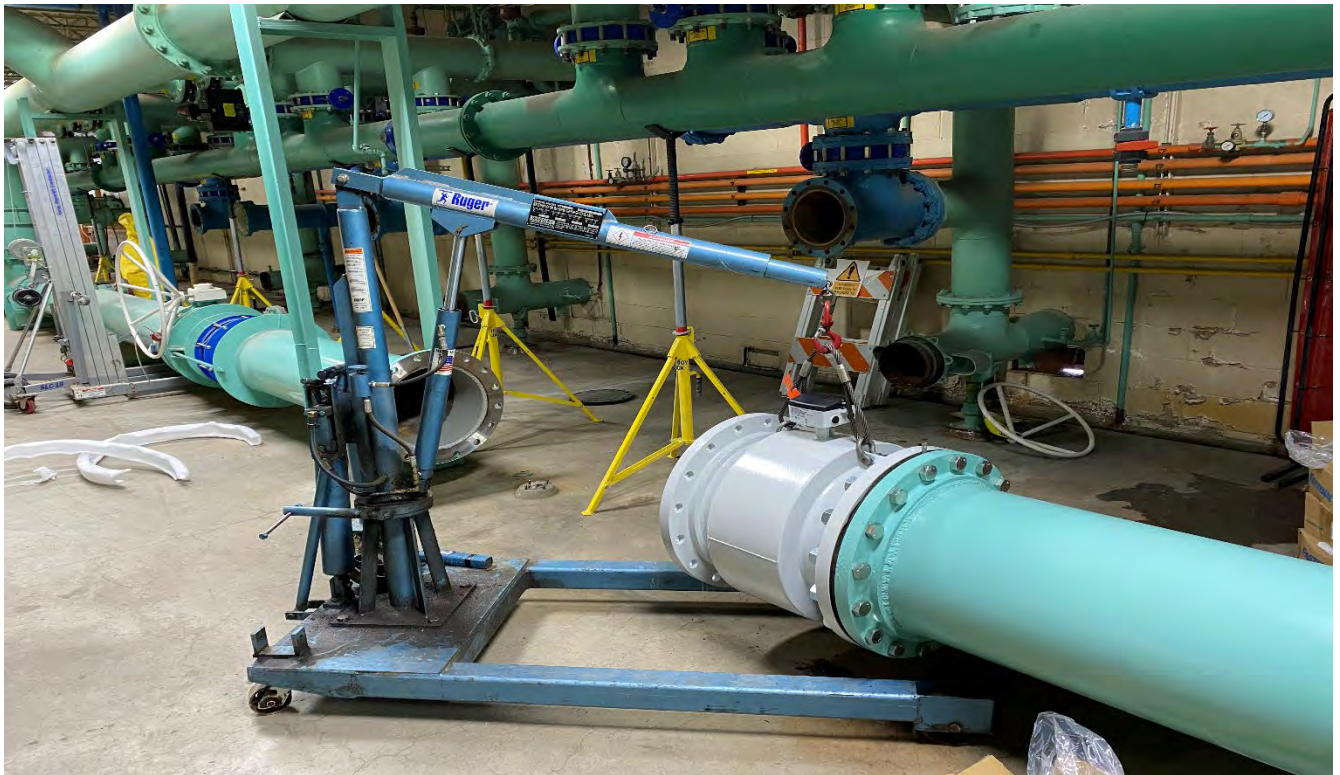
Final Effluent Flow Meter Installation
