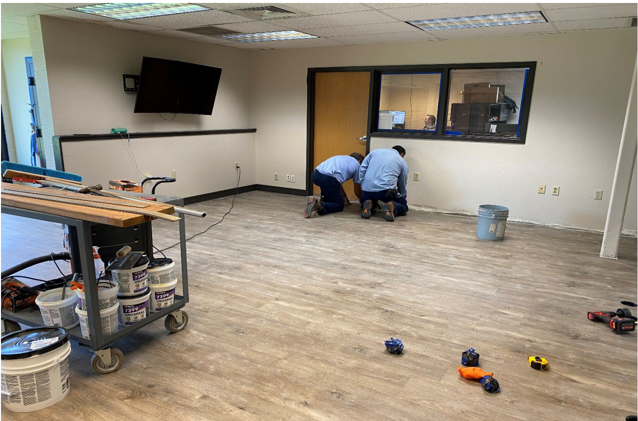
Maintenance Office Remodel
