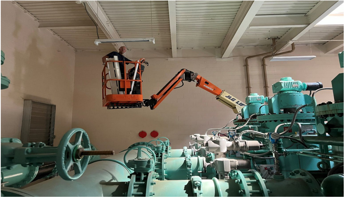
BNR Influent LED Light Upgrade
