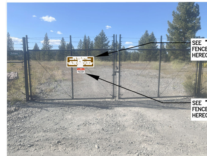
PHOTO 3 1. GATE LEADING TO THE LAY DOWN YARD, FACING WEST.
