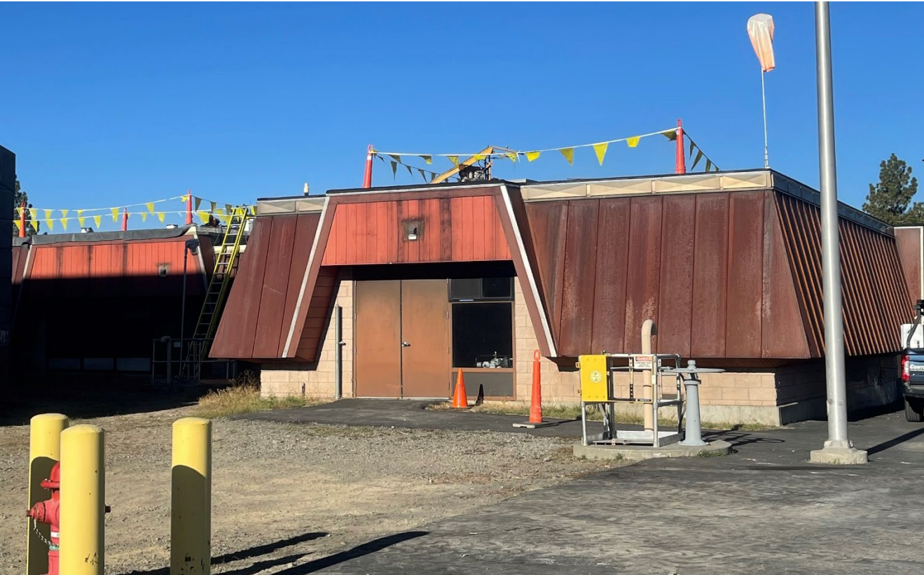
Building 24 – Roof Replacement
