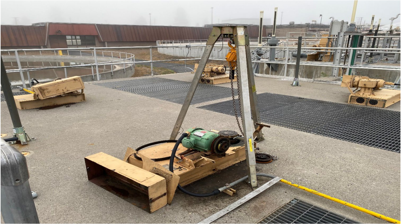
Flucculation Mixer Repair
