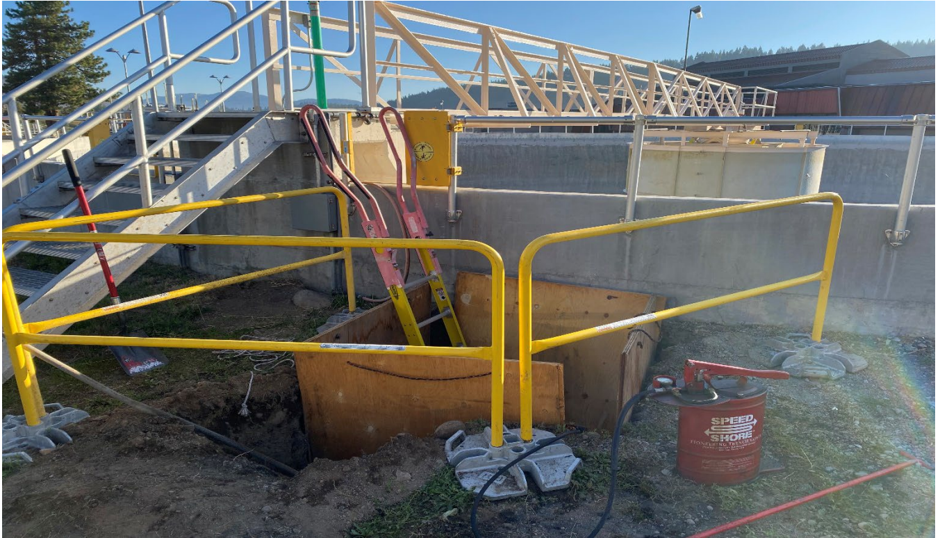
Two-water Yard Hydrant Repair at Secondary #2
