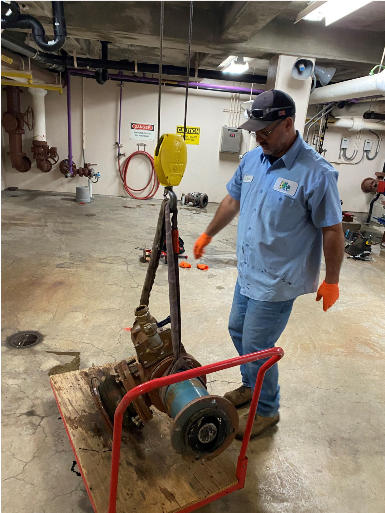
Digester #33 Transfer Pump Rebuild
