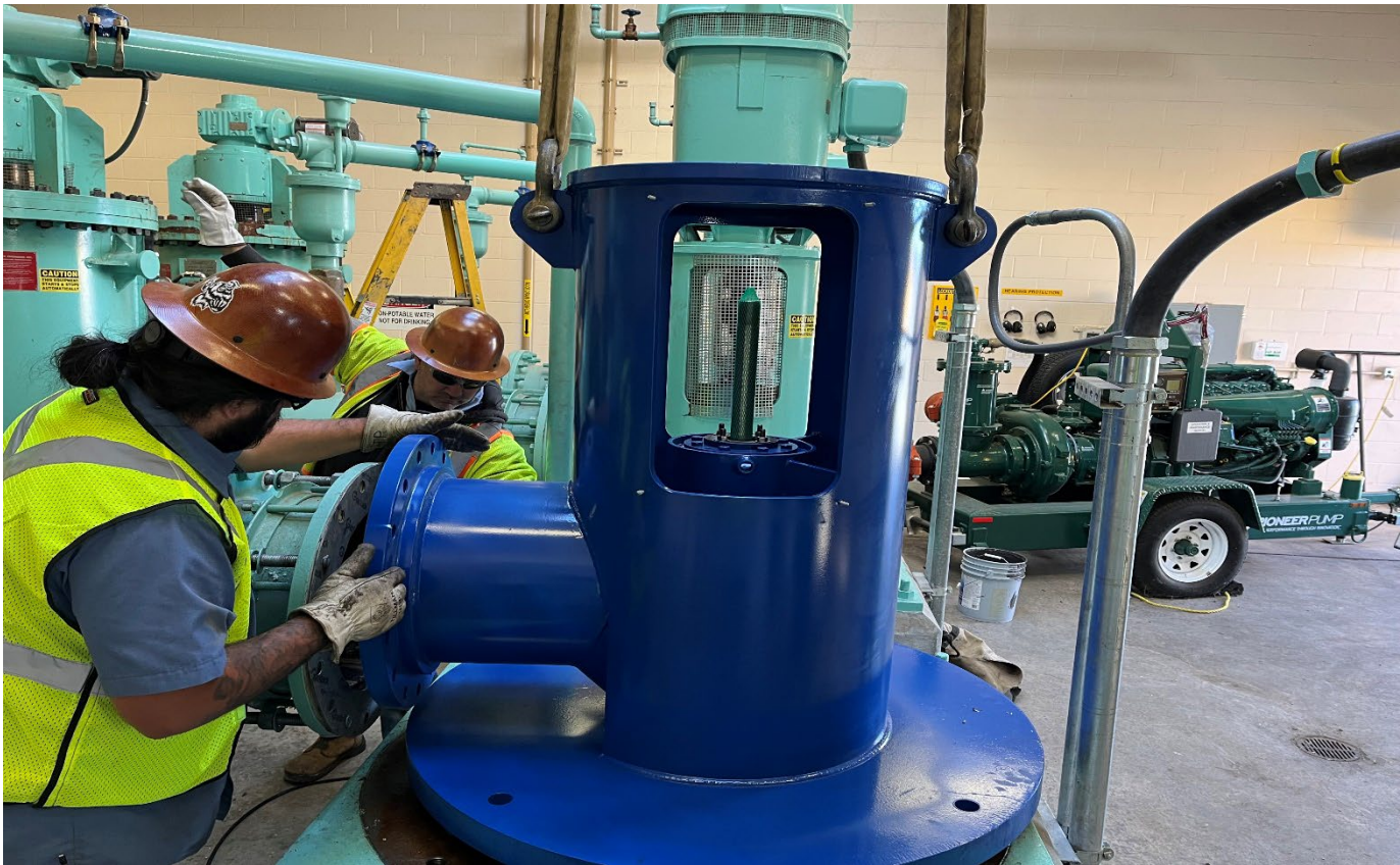
BNR Influent Pump Install
