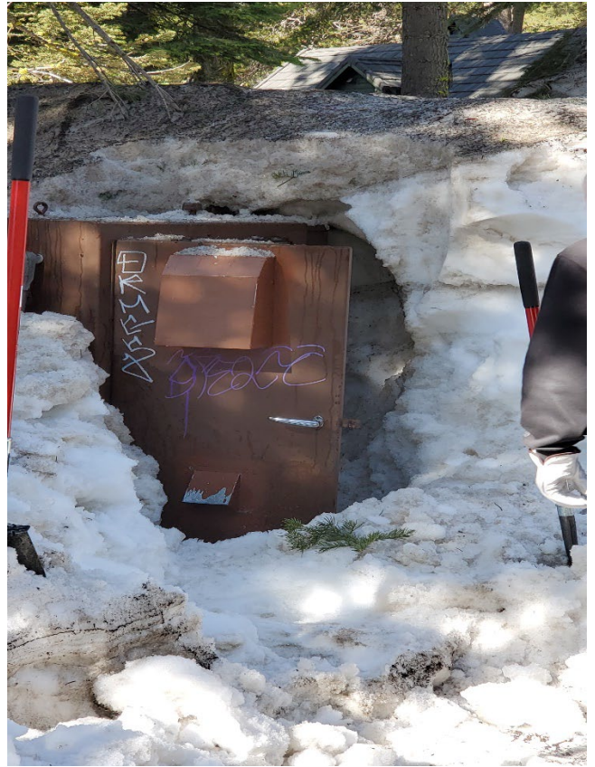
Ramparts Telemetry Vandalism
