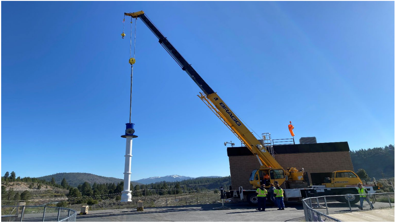
BNR Influent Pump Install
