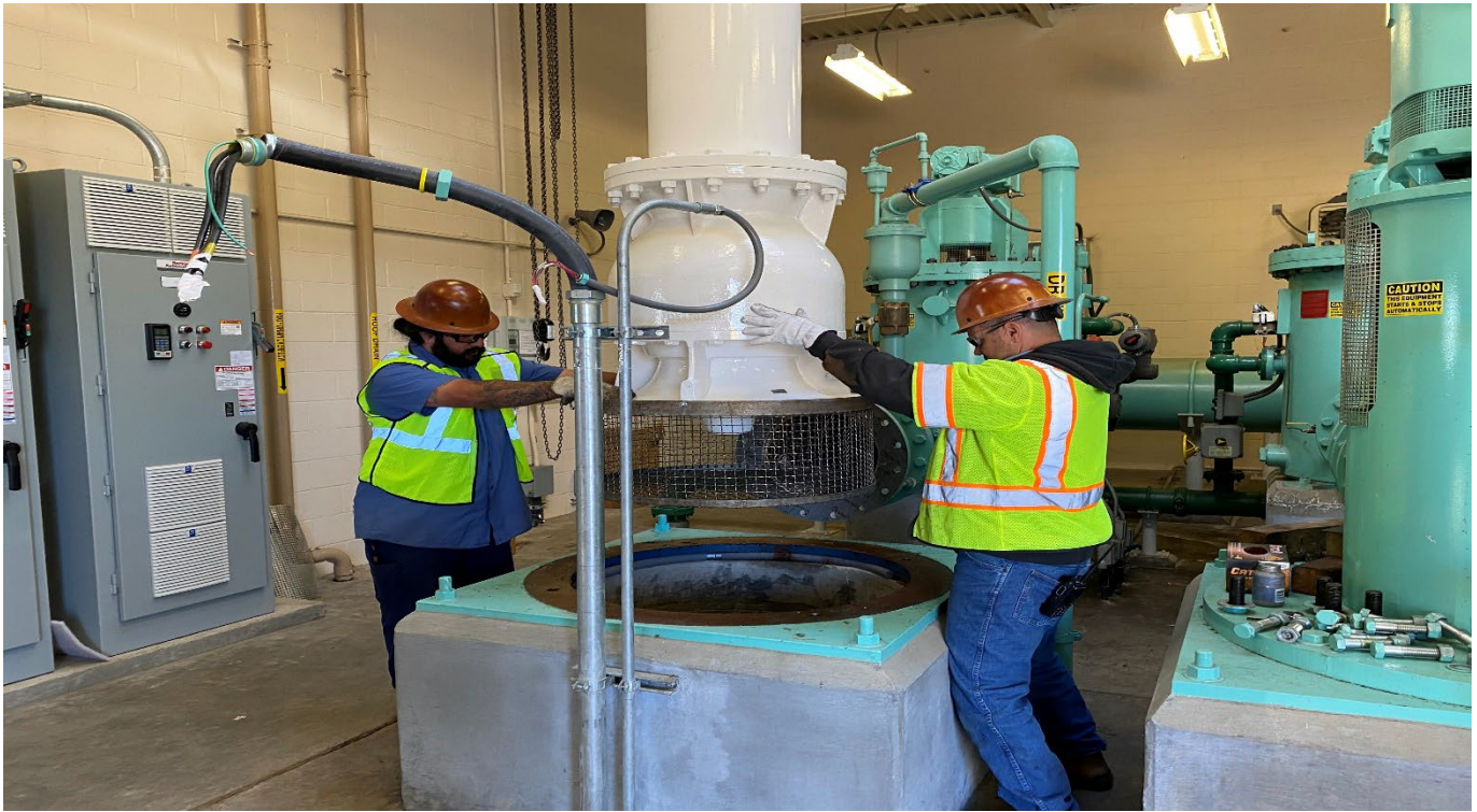
BNR Influent Pump Install
