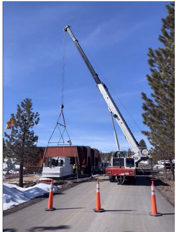
2021 Chlorine Scrubber Improvements Project Building 75-Installation of New Chlorine Scrubber
