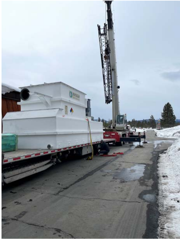
2021 Chlorine Scrubber Improvements Project Building 75-New Chlorine Scrubber Delivery
