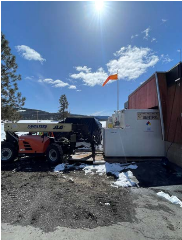
2021 Chlorine Scrubber Improvements Project Building 75-Removal of Existing Scrubber
