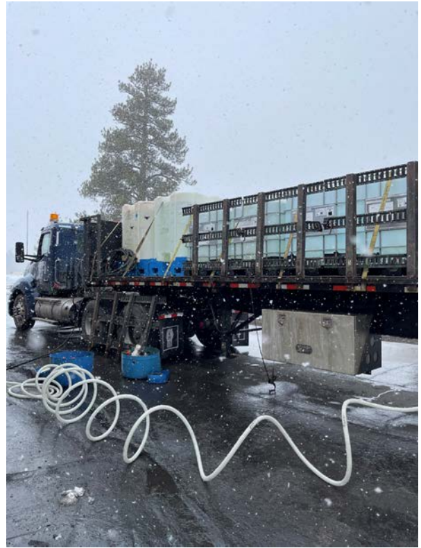
2021 Chlorine Scrubber Improvements Project Building 75-Removal of Chemical from Existing Scrubber
