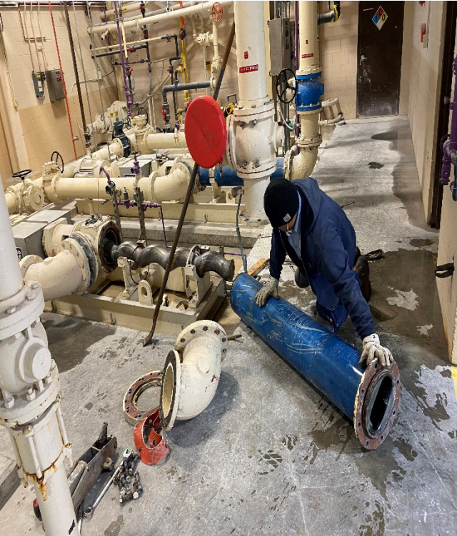
Filter Press Feed Pump Rebuild
