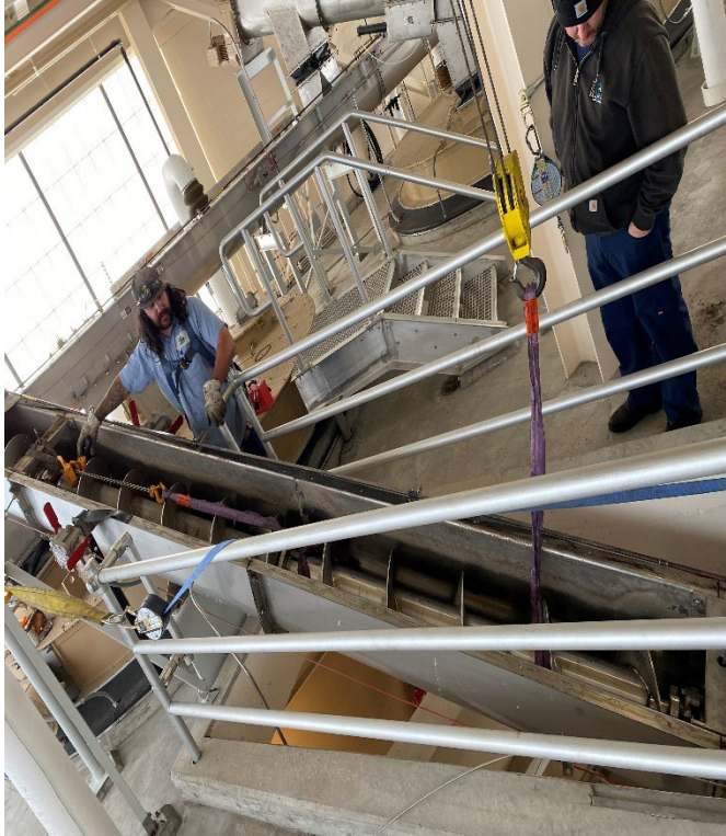
Cake Conveyor Repair
